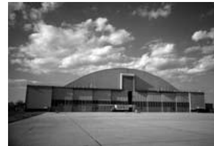
FIG. 9: Hangar #3, Andrews AFB, Maryland.
