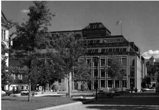
FIG. 11: Bank of Norway Head Office, façade as realized
