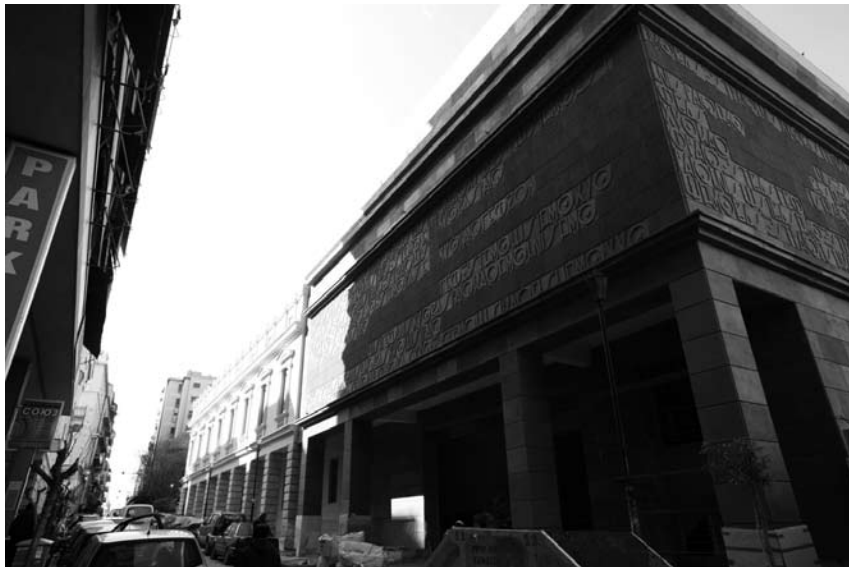
FIG. 1. Extension of the building of the National Theatre.
