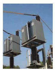
Figure 3.3: Voltage Transformer
