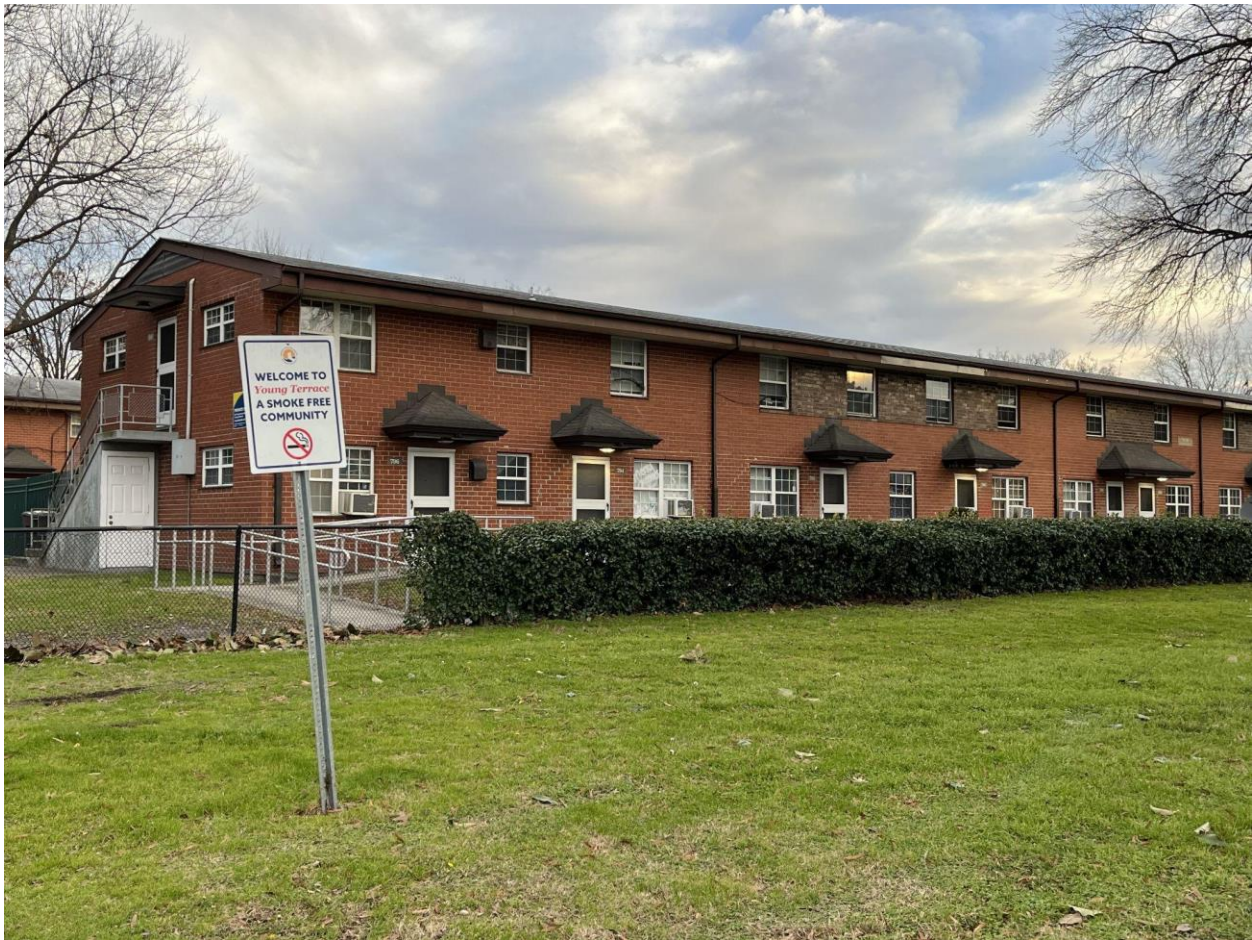
Figure 13: A public housing complex located at Young Terrace. Taken by Molly Frey, January 10, 2023.
