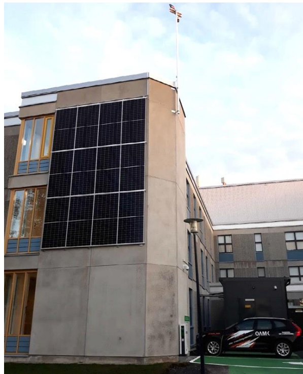
Figure 17: South wall vertical panels
