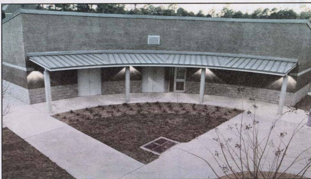
Construction is nearly complete for the new photo lab behind the Fine Arts Center. The new building will be 6,000 square-feet and will be able to handle more students than the current photo lab.
