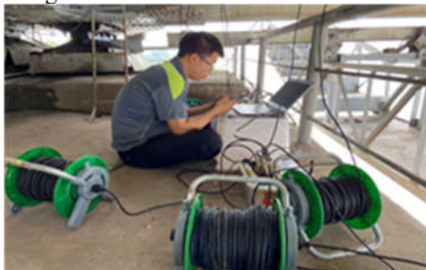
Fig. 7. Carry out direct monitoring by vibration method
