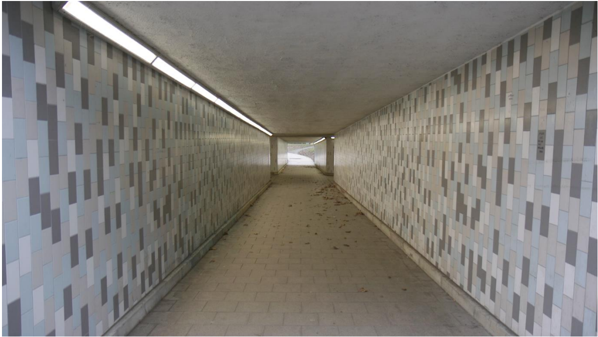
Figure 6.8 Tunnel toward Huddersfield town centre (Deep depth of field).
