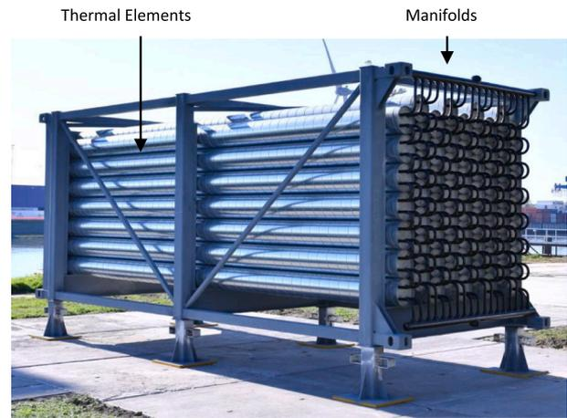
Fig. 3. Masdar Institute's concrete-based modular heat storage system.
