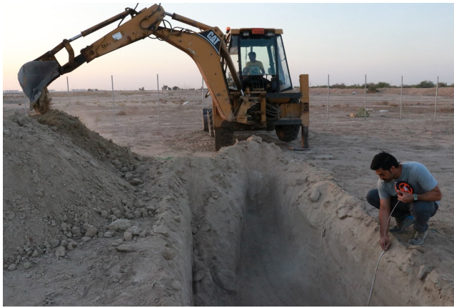
FIGURE 2 The grave's depth was checked using a measuring tape while digging the mass grave by the backhoe loader.
