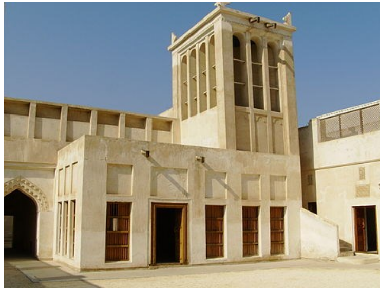
Figure 2.1: Use of natural ventilation in the Middle East (Isa bin Ali: Wikipedia)
