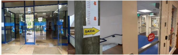
Fig. 2 - – Identification of the entrance door with the signs referring to the procedures in case of suspicion of COVID 19 (Cristina, 2021) a); Exit port identification, in Portugal and the United States of America (Cristina, 2021) b).
