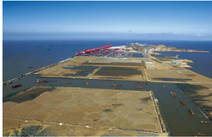
Figure 3.2 Land reclamation of Yangshan deep-water port (YH, 2007)
