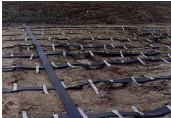
Figure 3.5 Horizontal drains in the transverse and longitudinal direction (Rujikiatkamjorn, 2005)
