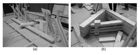
Figure 14. Making the plaza structure: (a) the working platform, and (b) the arrangement of timber boards.
