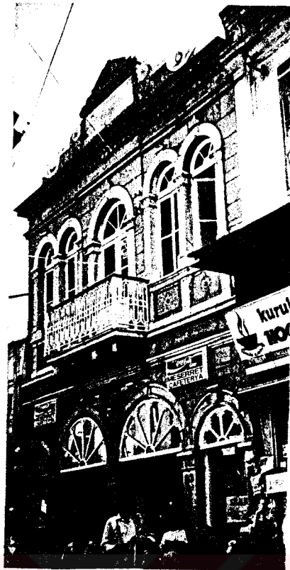
Figure 303 Meserret Hotel (Meserret Bazaar) after restoration, a view from Anafartalar Street (Hükümet Street)
