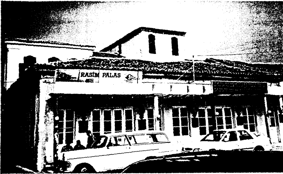
Figure 160 Rasim Palace Hotel, a view from the entrance side
