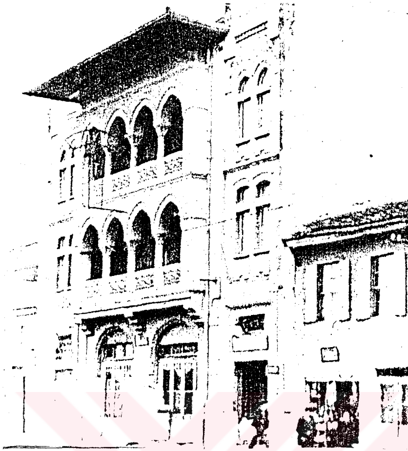
Figure 362 Bahçeli Hotel, a view from Gaziler Street prior to its demolition in 1986 (Archive of İzmir Conservation Council of Cultural and Natural Entities, Numbered 1)
