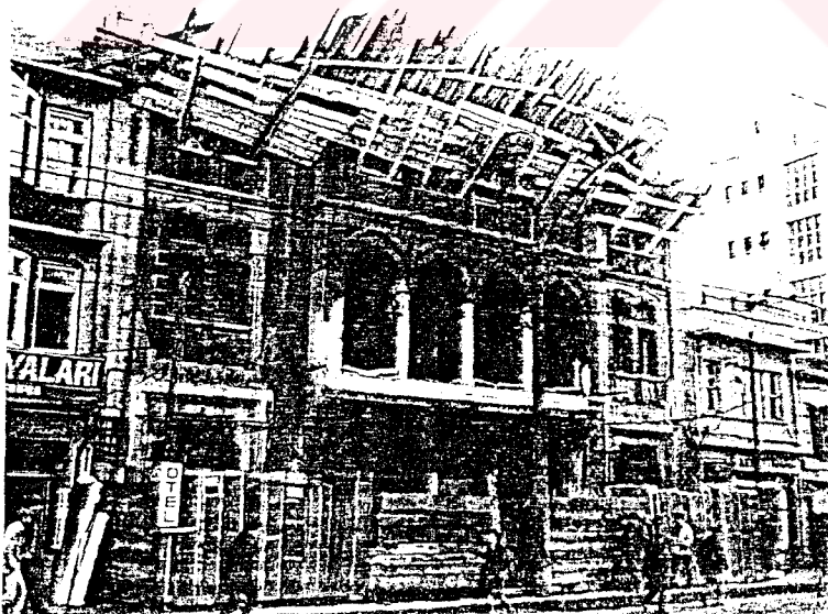
Figure 363 A photograph showing the demolition of Bahçeli Hotel (Archive of İzmir Conservation Council of Cultural and Natural Entities, Numbered 1)
