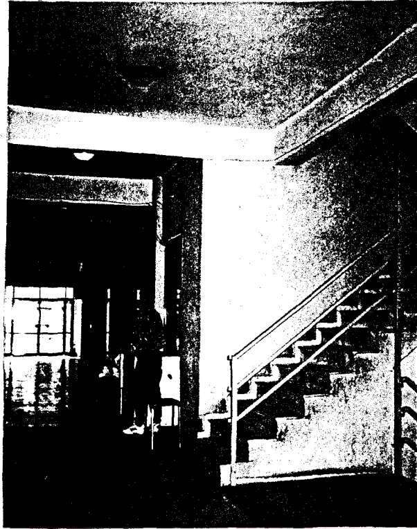
Figure 370 Bahçeli Hotel (Bahçeli Business Center) after restoration, the entrance hall and the stairs
