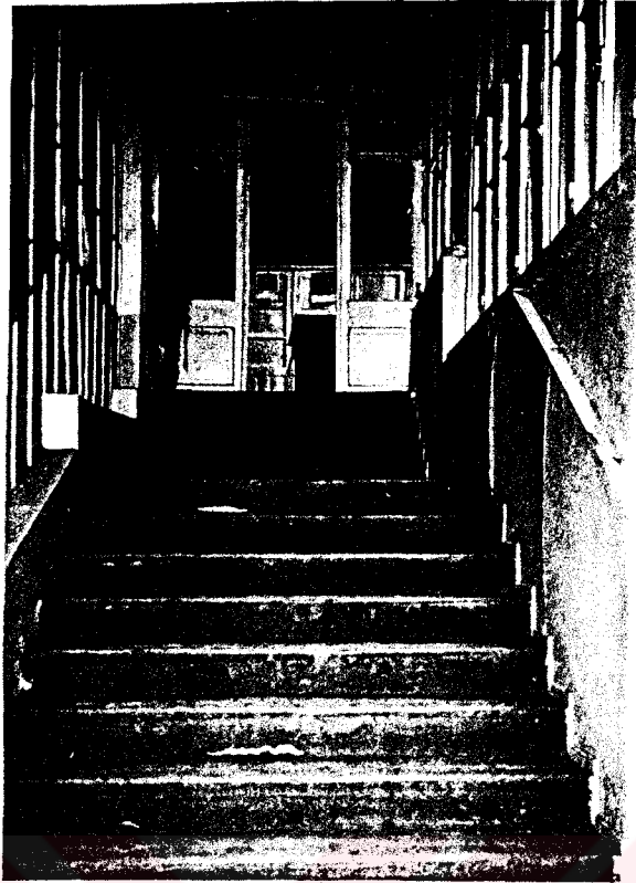
Figure 334 Sadık Bey (Yeni Sadık Bey) Hotel, the stairs at the entrance from Basmahane Square up to the hotel hall
