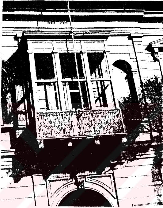
Figure 329 Naim Palace Hotel (Atatürk Museum), oriel placed above the entrance
