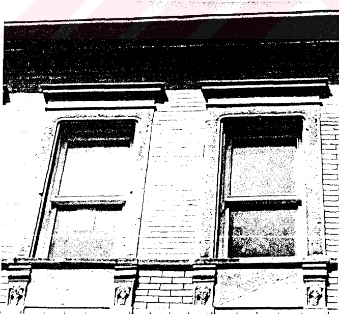
Figure 321 Ragıp Pasha Hotel (Ragıp Pasha Bazaar) after restoration, the windows of the first floor
