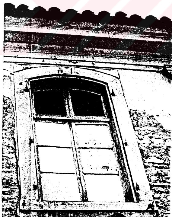
Figure 278 Hadji Sadullah Hotel, one of the upper floor windows facing the Veysel Cul-de-sac.
