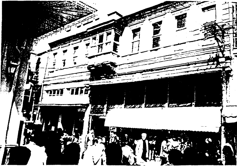
Figure 313 Ragıp Pasha Hotel, a view from Anafartalar Street (Hükümet Street) prior to restoration (Archive of İzmir Conservation Council of Cultural and Natural Entities, Numbered 1)
