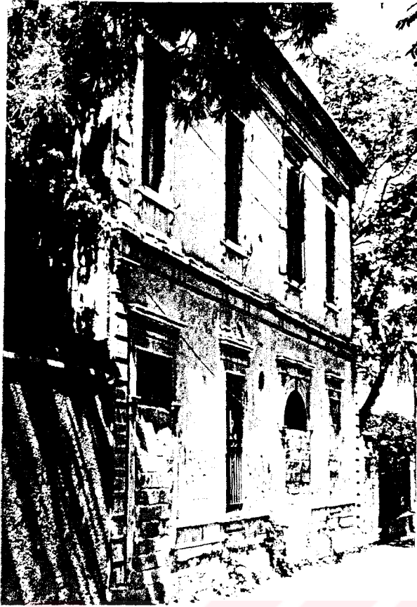
Figure 156 Manol Hotel - Buca, a view from the entrance side
