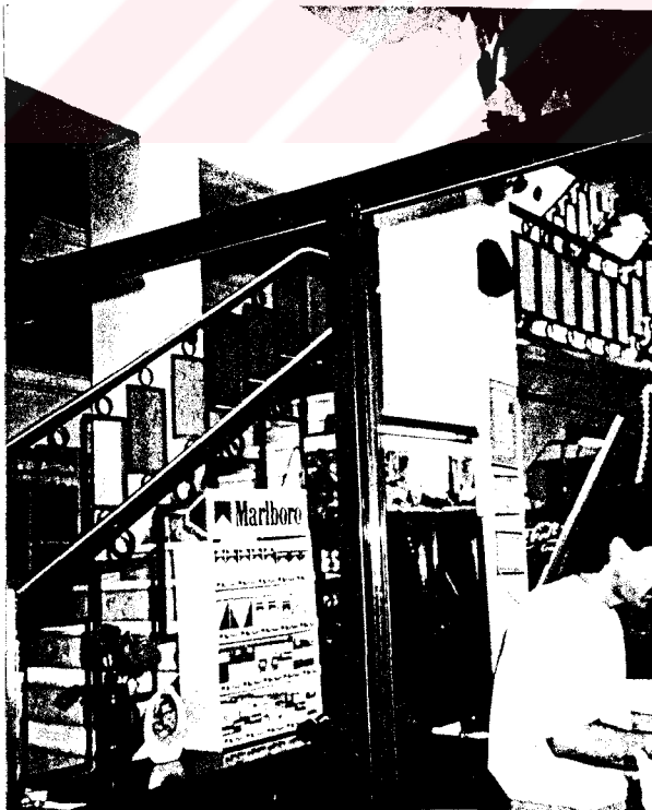
Figure 302 Meserret Hotel (Meserret Bazaar) after restoration, the stairs
