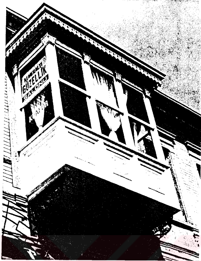
Figure 320 Ragıp Pasha Hotel (Ragıp Pasha Bazaar) after restoration, oriel of the first floor
