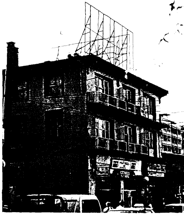
Figure 330 Sadik Bey (Yeni Sadik Bey) Hotel, the new section facing the Basmahane Square
