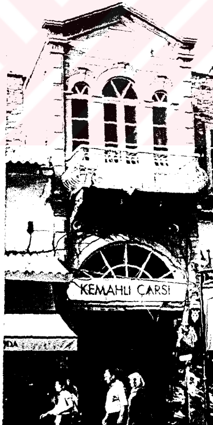
Figure 291 Kemahli (Kemahli İbrahim Bey) Hotel after restoration (Kemahli Bazaar), the view of the entrance
