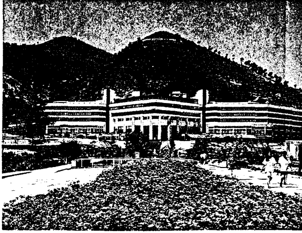
Figure 416 Princess Hotel, Balçova
