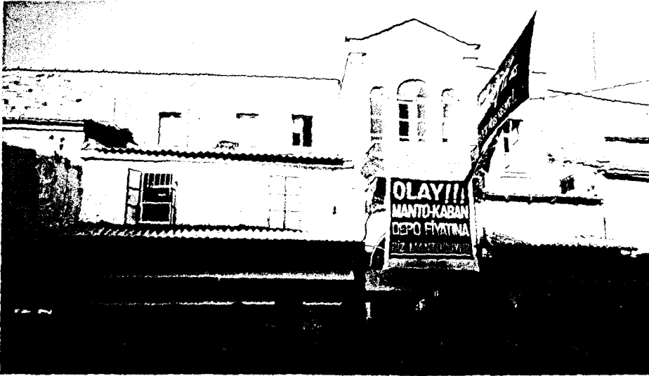
Figure 290 Kemahli (Kemahli İbrahim Bey) Hotel after restoration (Kemahli Bazaar), a view from Anafartalar Street (Kemeraltı Street)
