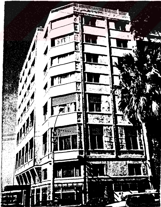
Figure 399 Kilim Hotel, Kazım Dirik Street
