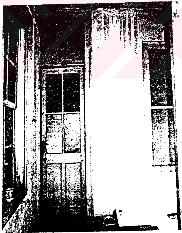
Figure 311 Ragıp Pasha Hotel, views from the corridors of the first floor prior to restoration (Archive of İzmir Conservation Council of Cultural and Natural Entities, Numbered 1)
