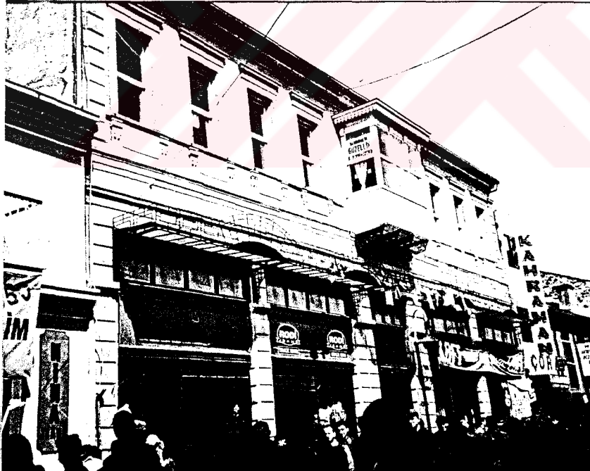
Figure 319 Ragıp Pasha Hotel (Ragıp Pasha Bazaar) after restoration, a view from Anafartalar Street (Hükümet Street)
