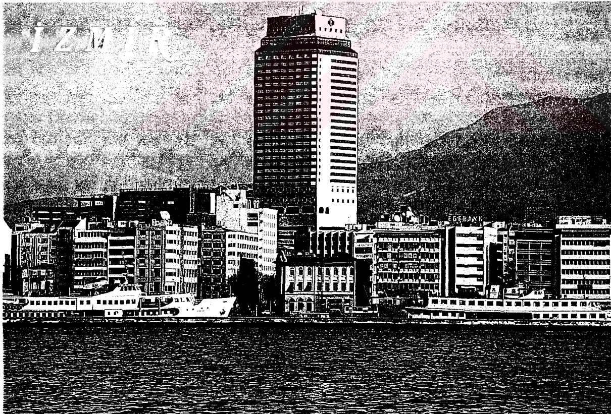
Figure 413 In a recent postcard, the new landmark as Hilton Hotel (as a skyscraper)
