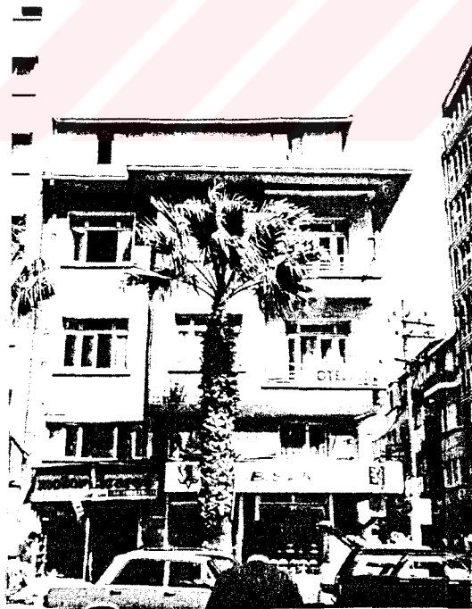
Figure 397 Uşak-Kervan Hotel, Fevzipasha Boulevard
