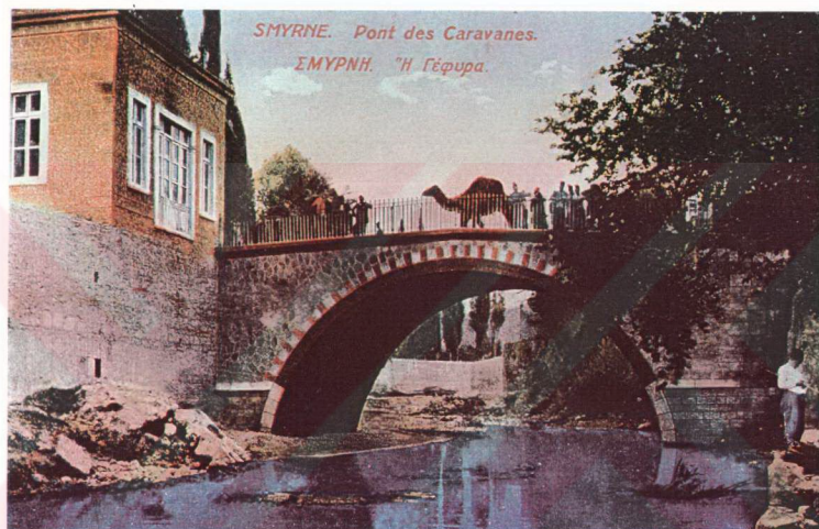
Figure 101 The Caravans Bridge from an old photograph
