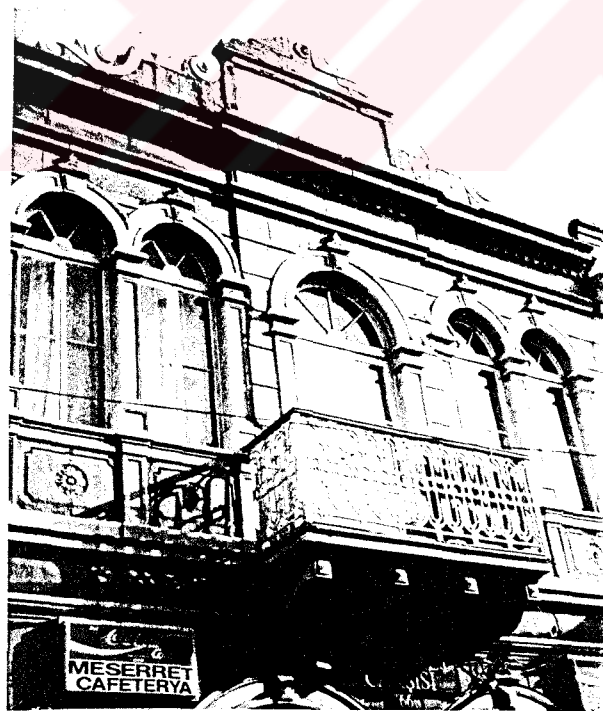
Figure 304 Meserret Hotel (Meserret Bazaar) after restoration, the balcony and the upper floor
