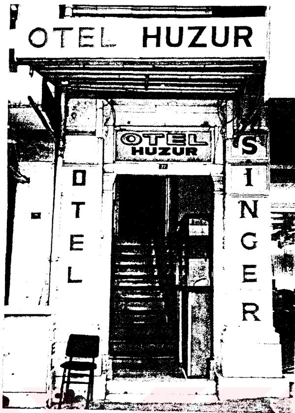
Figure 349 Aydin-Kasaba (Huzur) Hotel, the entrance door
