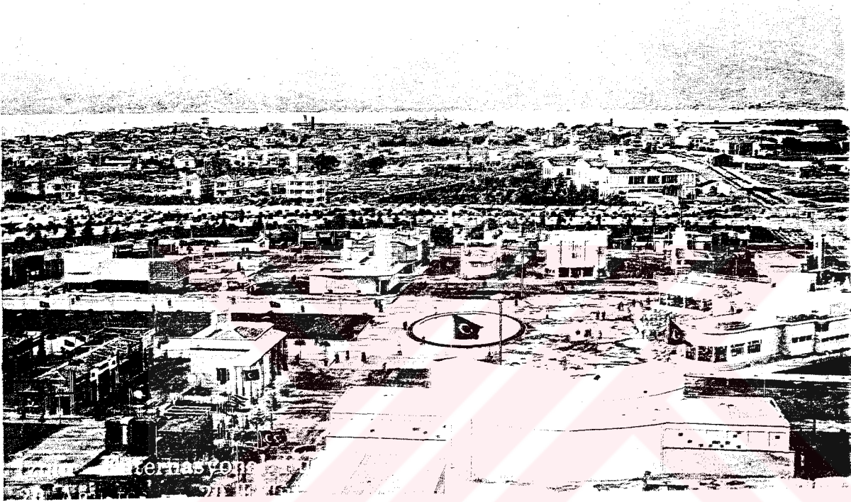
Figure 115 International Fair of Izmir and the renewed city of Izmir
