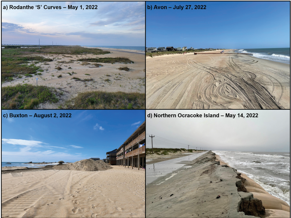
Figure 5. Photographs of recent coastal adaptation and mitigation actions at the Seashore: A) Rodanthe Bridge (aka the “Jug Handle” bridge) illustrates adaptation by relocation to avoid overwash; B) beach nourishment at Avon and C) Buxton represents short-term mitigation of frequent ocean overwash of NC 12; D) sandbags installed along the northern section of Ocracoke Island are intended as a temporary mitigation response to rapid erosion while various sites are under consideration for the relocation of the South Dock ferry terminal (Photo Credit: Cape Hatteras National Seashore, National Park Service [2021]).
