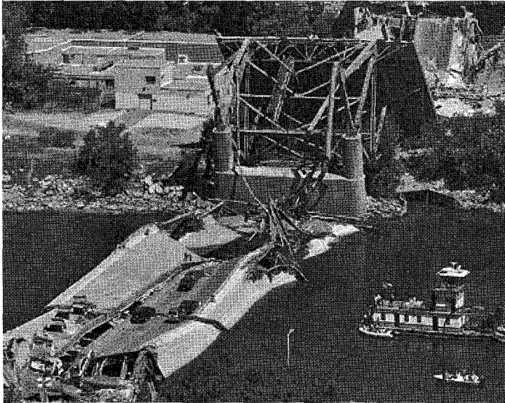
Figure 2: I-35W Bridge collapse in Minneapolis, Minnesota on August 2, 2007. 40
