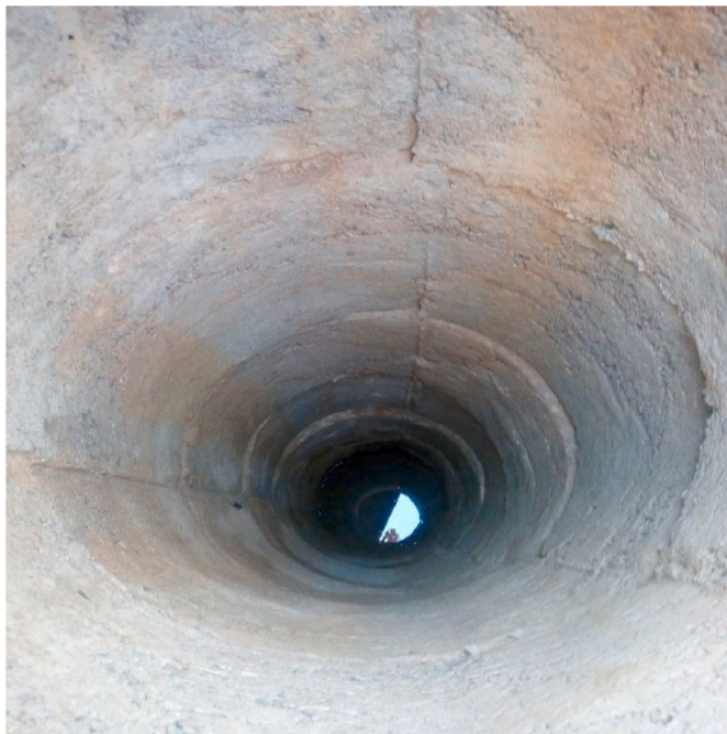
Fig. 2. Showing un-screened concrete-lined large-diameter hand-dug well.
