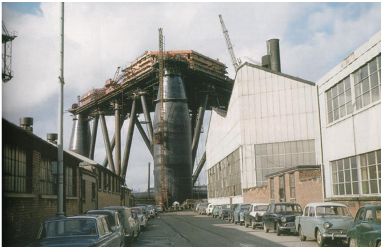
The Sea Quest under construction at Harland & Wolff Construction Company in 1966. According to Harland & Wolff, “the entire structure was 320 feet (98 m) high and weighed 150,000 tons, including three legs each 35 feet (11 m) in diameter and 160 feet (49 m) long” (see fn 37 above).
