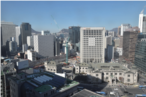
Figure IV- 5. Construction Site of Bank of Korea's Integrated Annex (as of January 2021)
