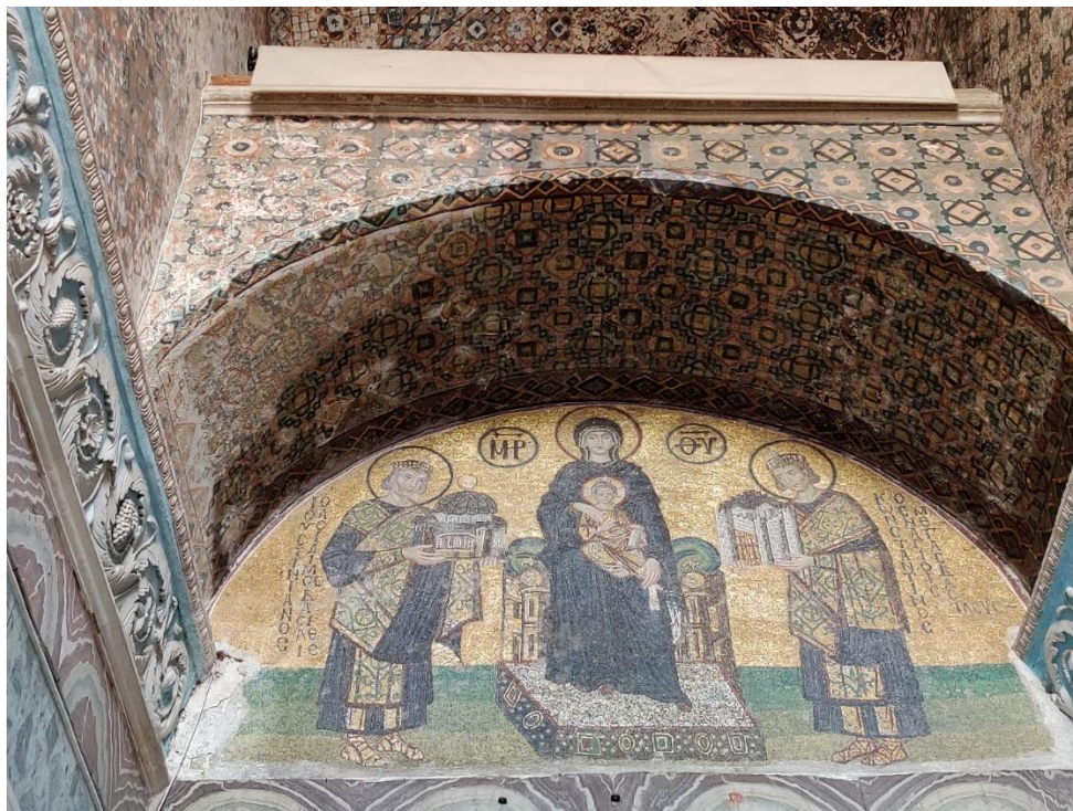
Figure 39: A rolled-up drape on a pulley system is located at the top of the tympanum, used to veil the mosaic in Hagia Sophia's vestibule (2021).
