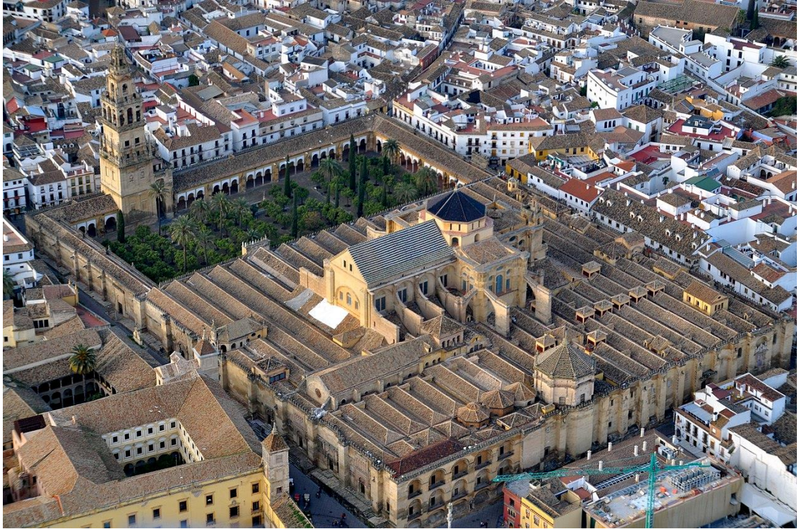
Figure 51: A cruciform Renaissance church was constructed into the former mosque of the Mosque-Cathedral. Source: Toni Castillo Quero.
