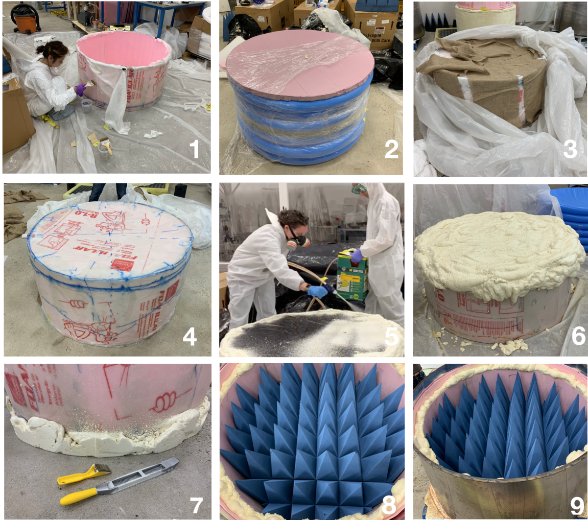
Figure 4.3: Foam and fiberglass insert construction procedure: (1) Laying down initial fiberglass cloth layers; (2) Inflatable tub used to keep insert shape during vacuum sealing; (3) fiberglass tub with peelply and burlap layers within an open vacuum bag; (4) fiberglass insert after vacuum bagging; (5) spray-foam procedure (photograph from earlier prototype); (6) spray polyurethane foam on base of insert; (7) leveling out foam on insert base; (8)(9) After filling in our remaining foam, we have an LN 2 -proof insert (subject to further testing), including the RF absorber for fit-checking.
