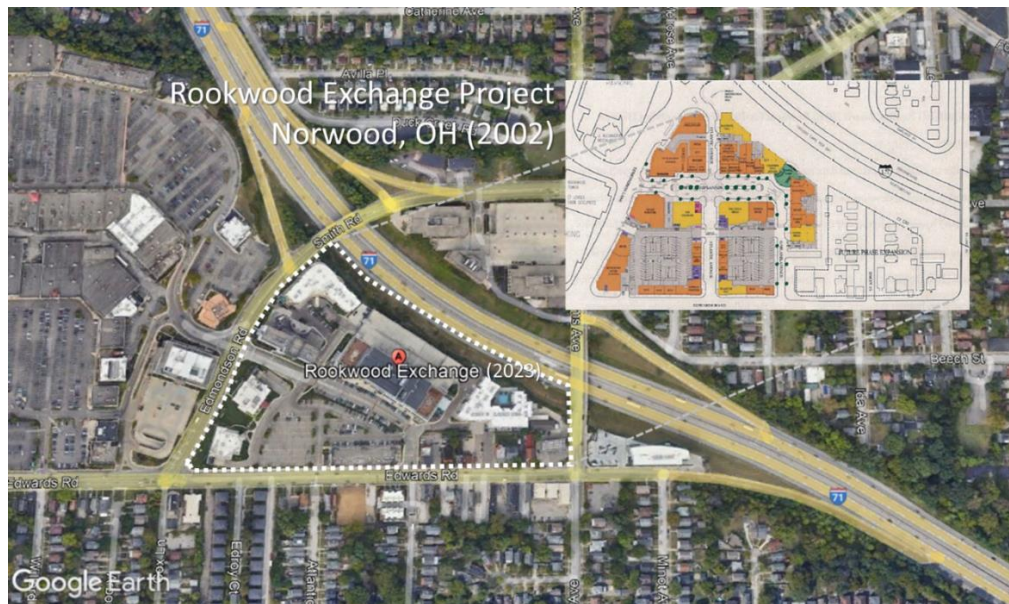
Figure 4.8 Rookwood Exchange Project Norwood, Ohio (2002)
