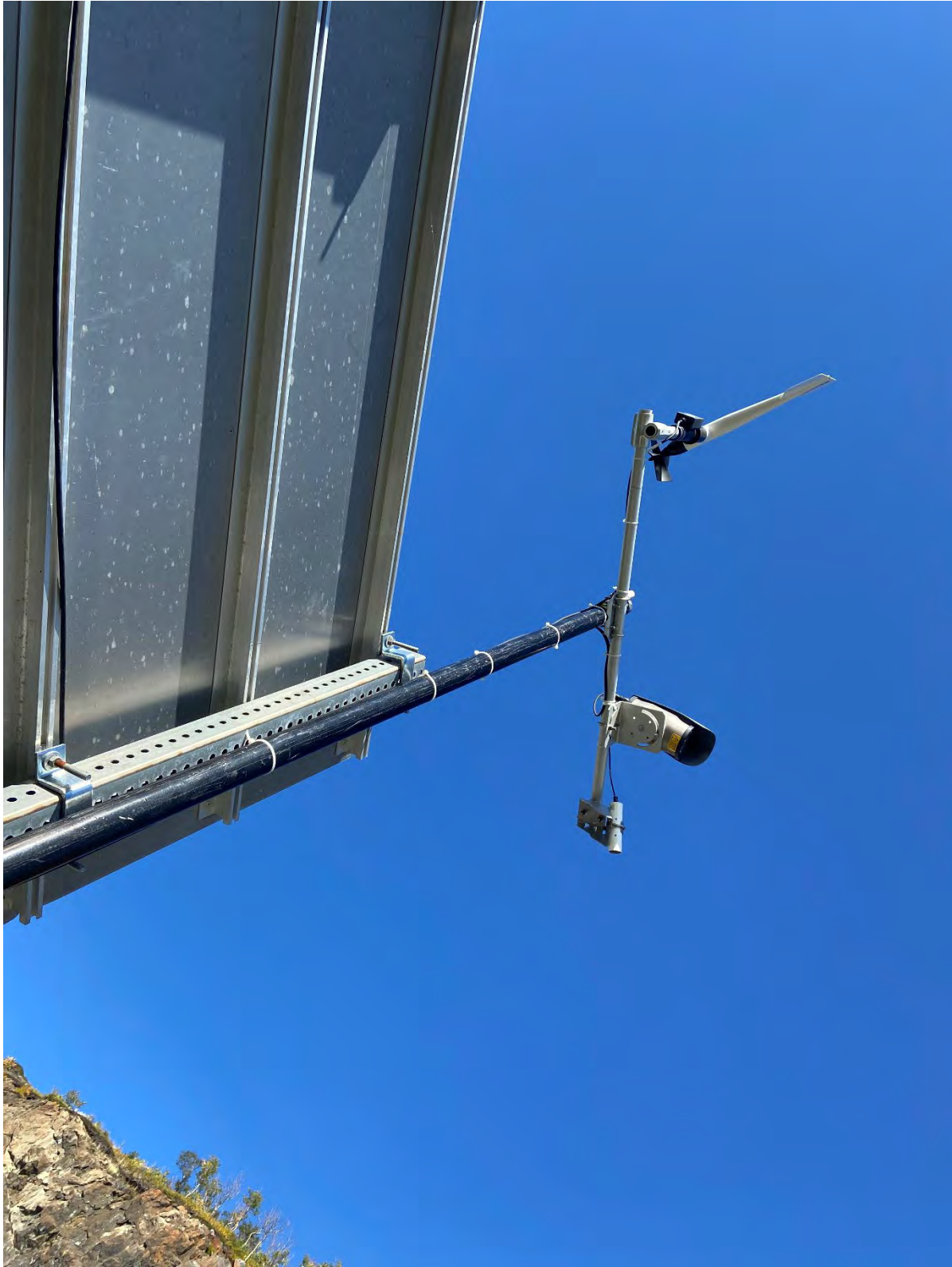
Seward Highway MP 113.5: Kalitec Post bolted to sign post.
