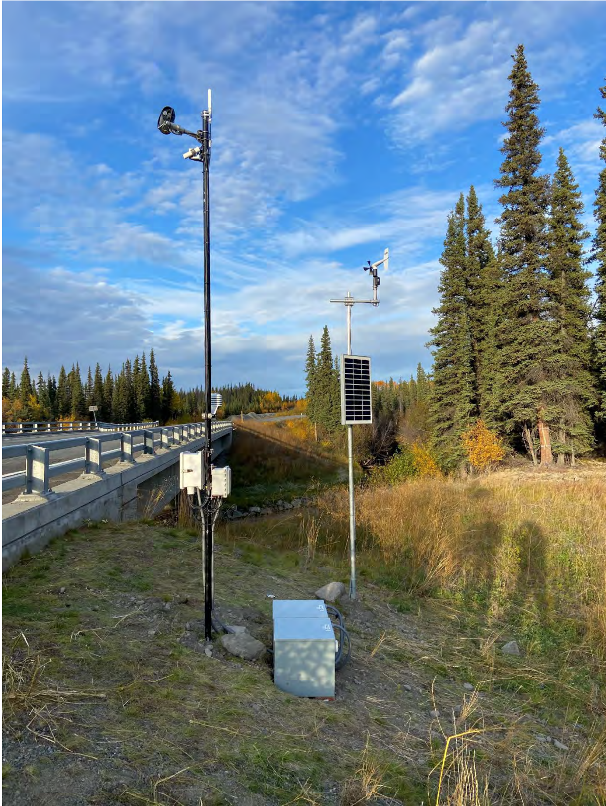
Tok Cutoff MP 17.5 view looking east toward Tulsona Creek.
