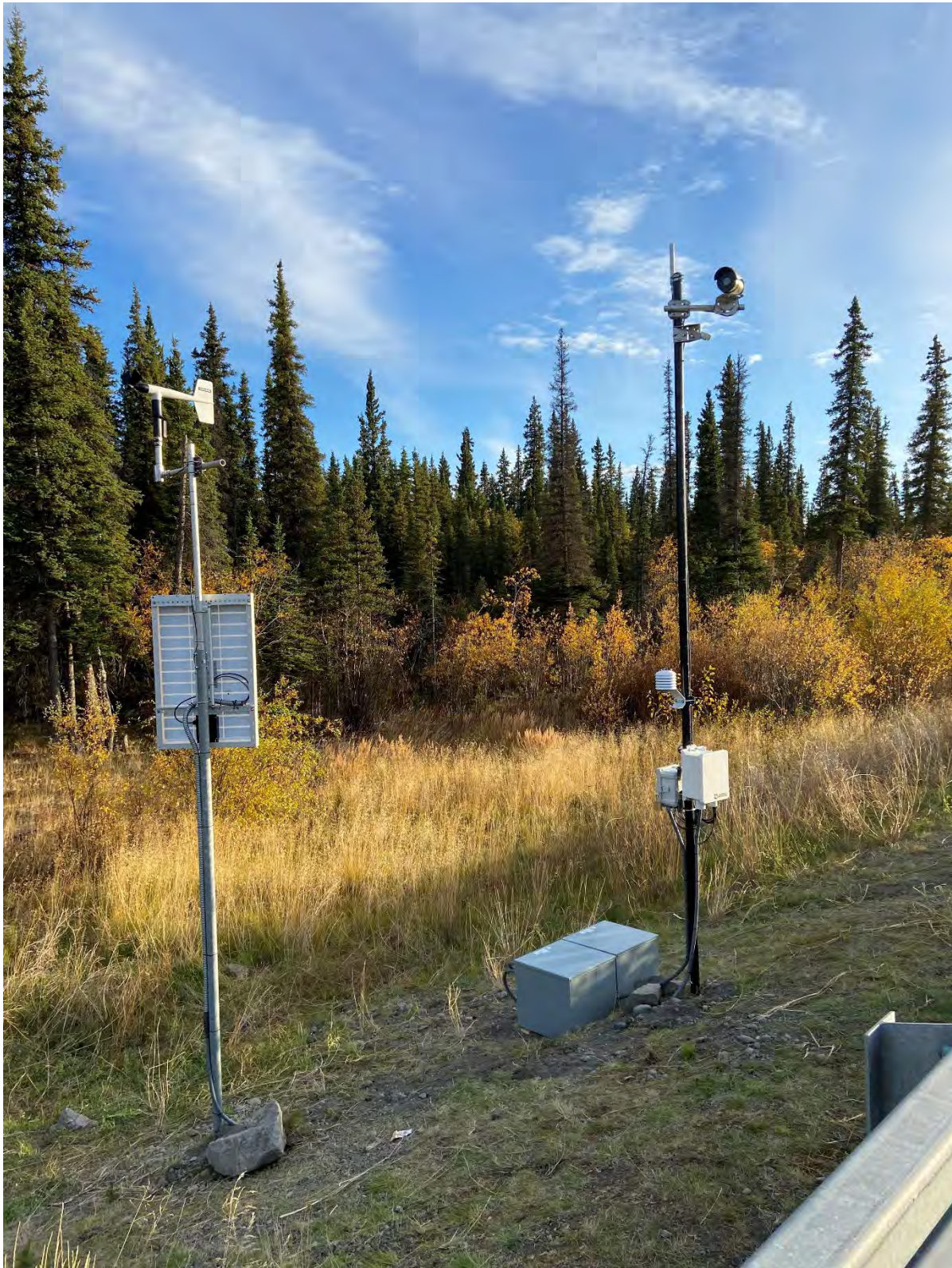
Tok Cutoff MP 17.5 view looking southwest from roadway.
