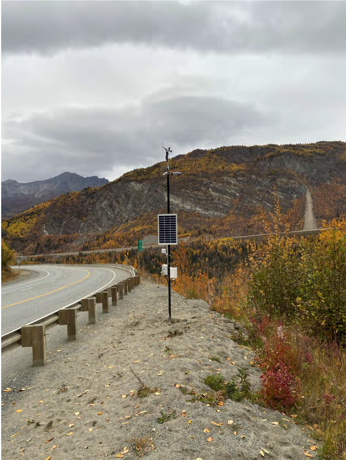
Glenn Highway MP 106 view looking north.
