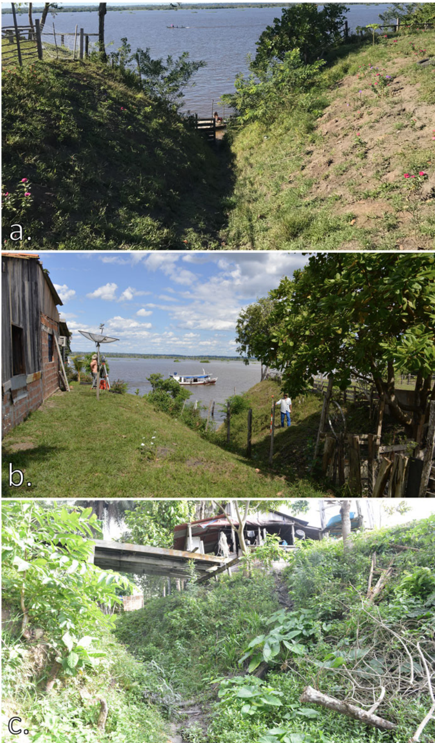
Figure 6. (a) Southeast view of Wharf 1 from lake bluff; (b) south view of Wharf 2 with house constructed on bluff; (c) north view of Wharf 3. (Photographs by Anna T. Browne Ribeiro.)
