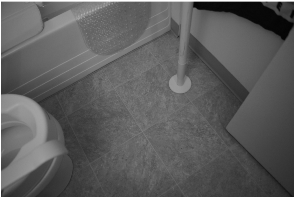
Figure 2: Suboptimal environment of case 3 when participating in bathing activity. Note. Adult with DMI was unable to get close enough to the bathtub with his wheelchair to transfer safely because of limited space, combined with placement of toilet and bathtub, and a floor-to-ceiling pole.
