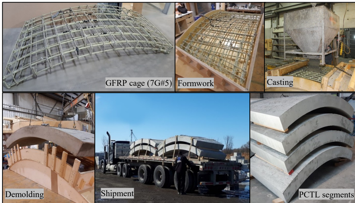
Figure 4.2 GFRP-reinforced tunnel segment cage and specimen fabrication.
