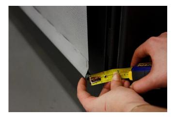
Figure 118. Measuring shading fabric distance
