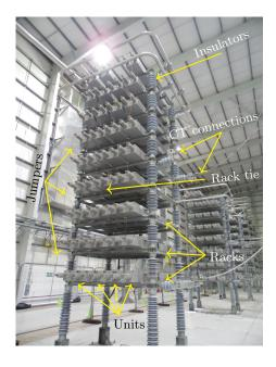
Figure 2.4: A large capacitor bank
