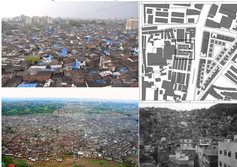
Figure III.19: Examples of building per site area assessment – building density – using aerial picture and site maps in slums. Upper-left is Dharavi, Mumbai 80 – high building density, upper-right is Haji Kasam Chawl, Mumbai 81 – standard building density, lower-left is Kibera, Nairobi 82 – high building density, lower-right is Rocinha, Brazil 83 – high building density.
