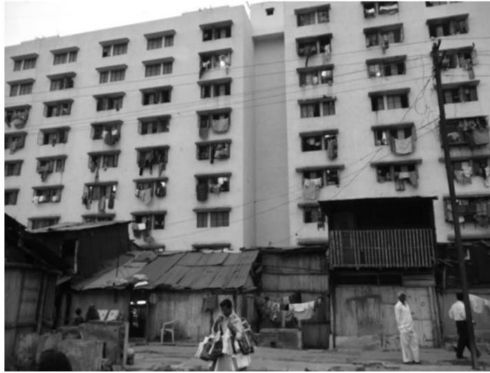
Figure III.12: Nanapeth re-housing project in Pune, India is deteriorating into slum. 41
