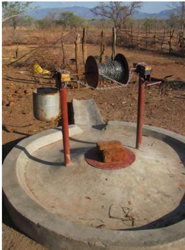
Figure III.15: A protected water well. Source: (UnitingWorld, n.d.).
