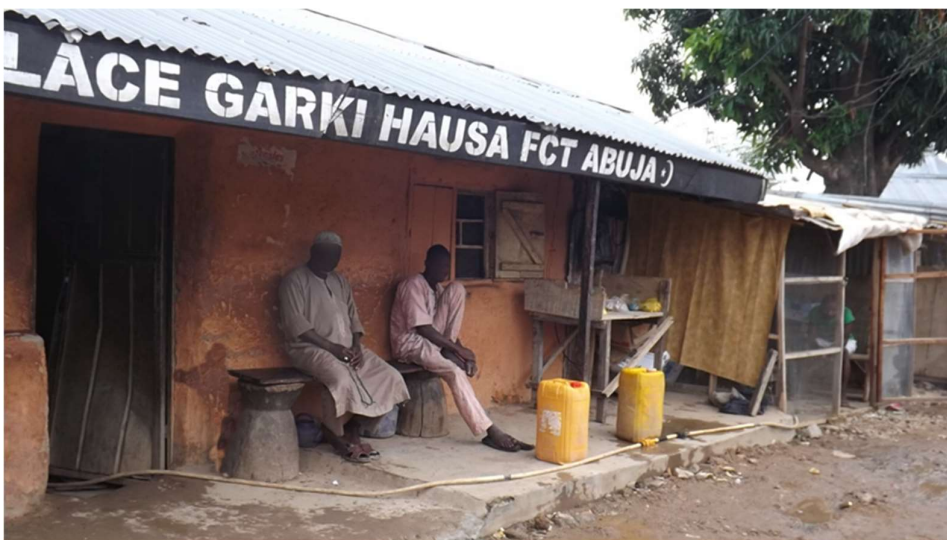
Figure 8.31: This building was upgraded from a 'daube' mud block with cement plaster. Source: author.
