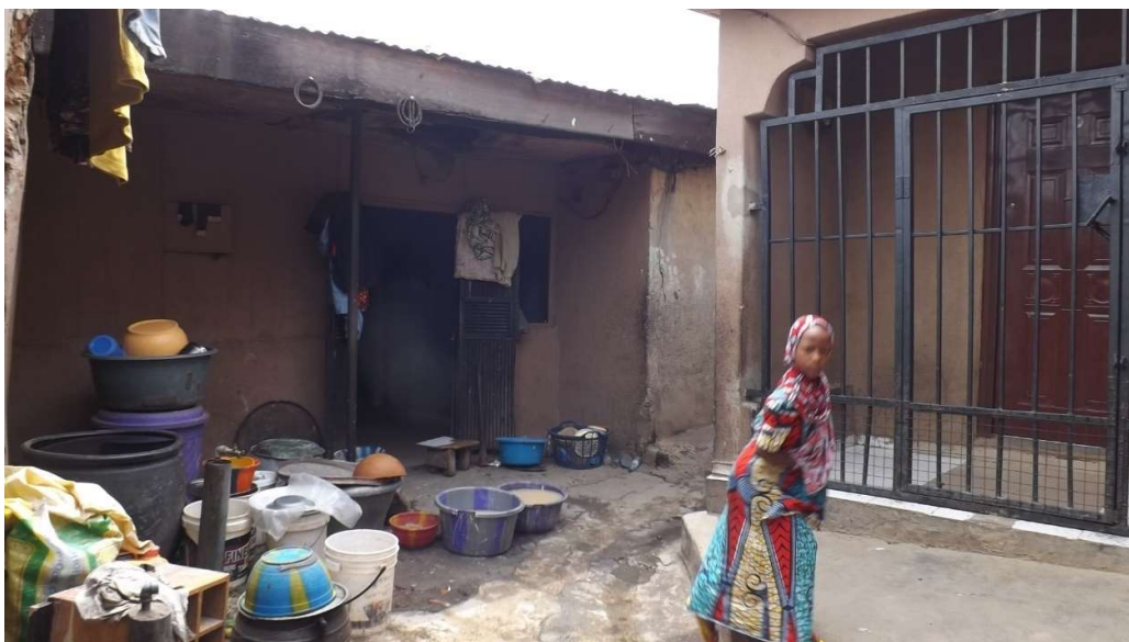
Figure 8.28: Recent building addition constructed of sandcrete block (on right). Source: author.
