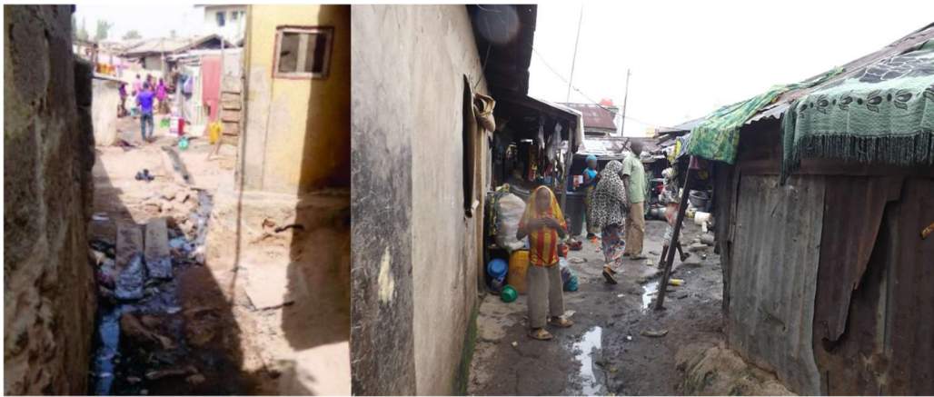
Figure 8.19: Household grey water forming open gutters in housing compounds. Source: (Image on left) (Itua et al., 2016), author.
