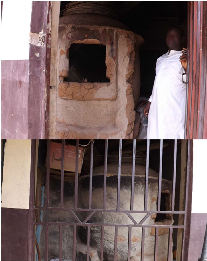
Figure 8.32: A house extension (sandcrete block construction) that creatively retains a traditional mud 'daube' grain silo in its design. Source: author.
