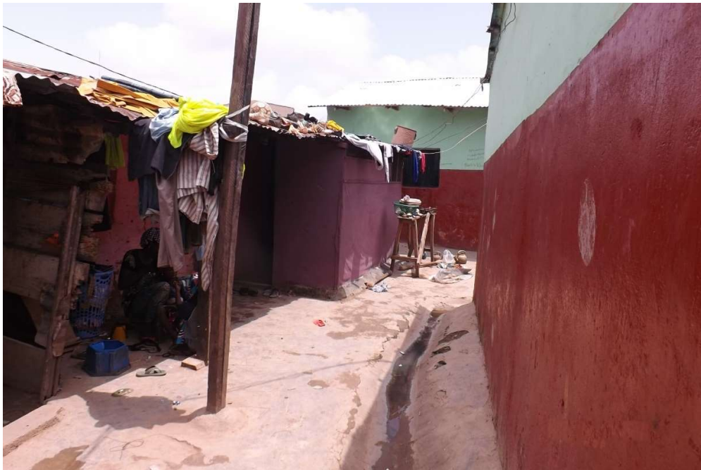
Figure 8.29: Building addition (on left) constructed from plywood to accommodate family growth, while the main building (on right) was incrementally upgraded to sandcrete structure. Source; author.
