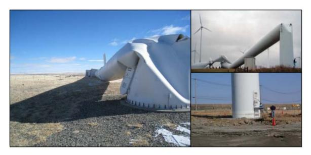
**Figure 1.2** Wind turbine collapse due to ground-shaking in Japan (left) and New Zealand (right). Taken from Asareh (2015).
