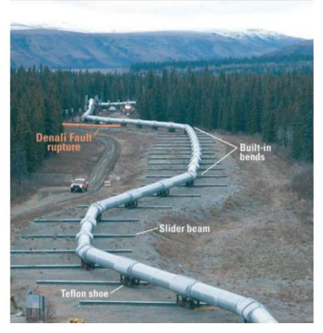
**Figure 1.3** Slider system for the Trans-Alaska pipeline and the horizontal displacement resulting from the 2002 Denali earthquake fault rupture. Taken from United States Geological Survey (2003).
