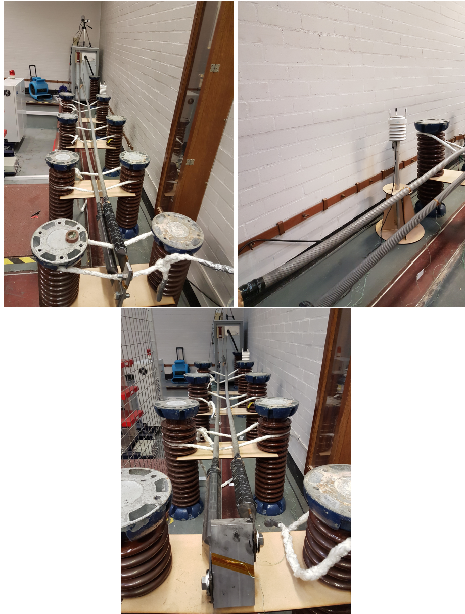
Figure 3.7: The overhead line experimental setup, including power supply, conductors, fan and weather station.
