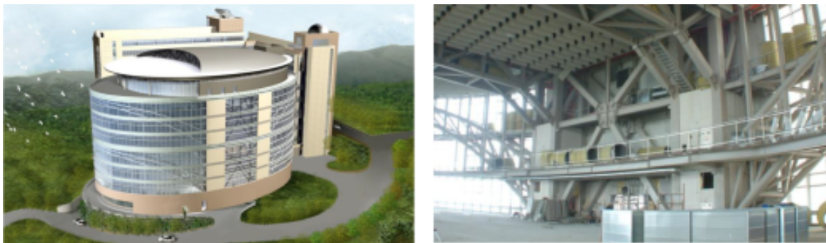
Figure 1.3: 10-storey gymnasium application at Chinese Culture University, Taipei from Lin et al. (2012)
