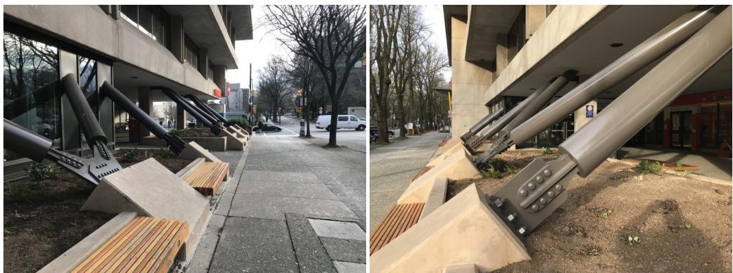
Figure 1.1: Vancouver City Hall, steel moment frame built in 1975 and retrofitted with 16 BRBs for earthquake demands in 2016. Image from: CoreBrace (2016)
