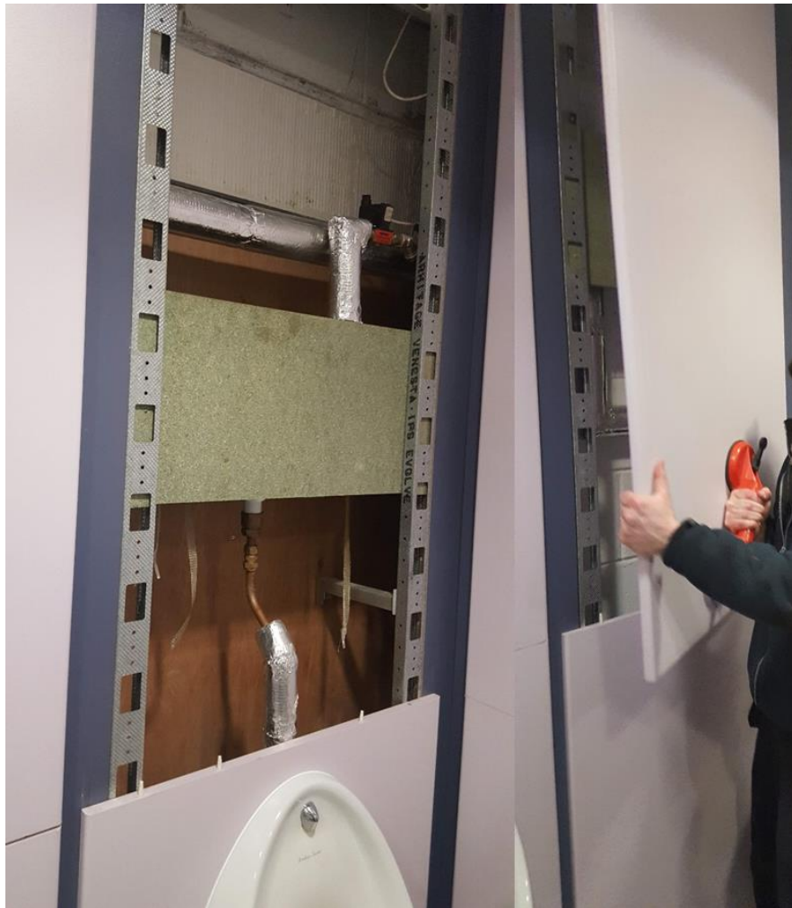
Figure 5-6 Removal of a wall panel by a plumber
