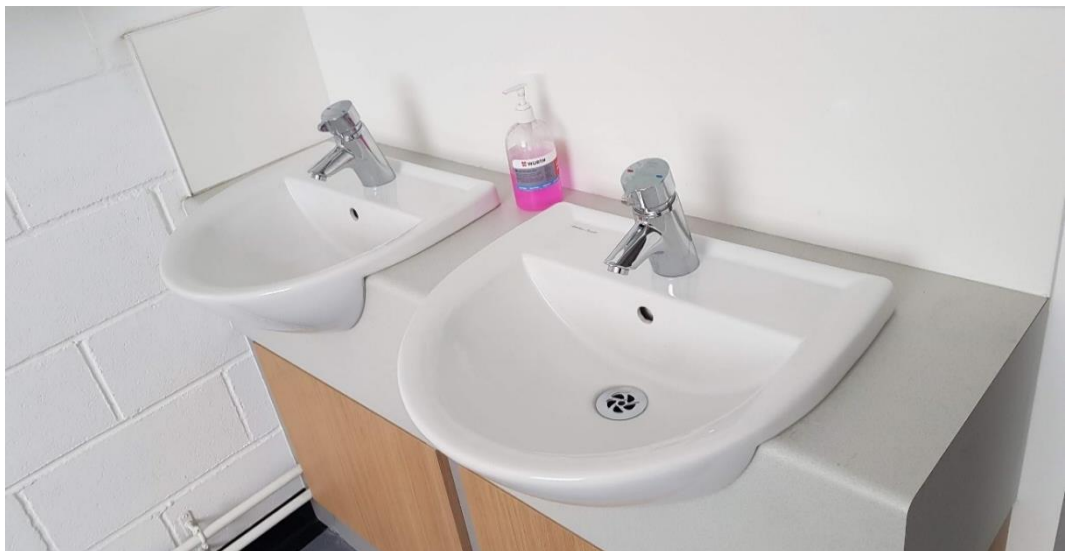
Figure 5-23 Self-closing water tap in the Postgraduate Centre
