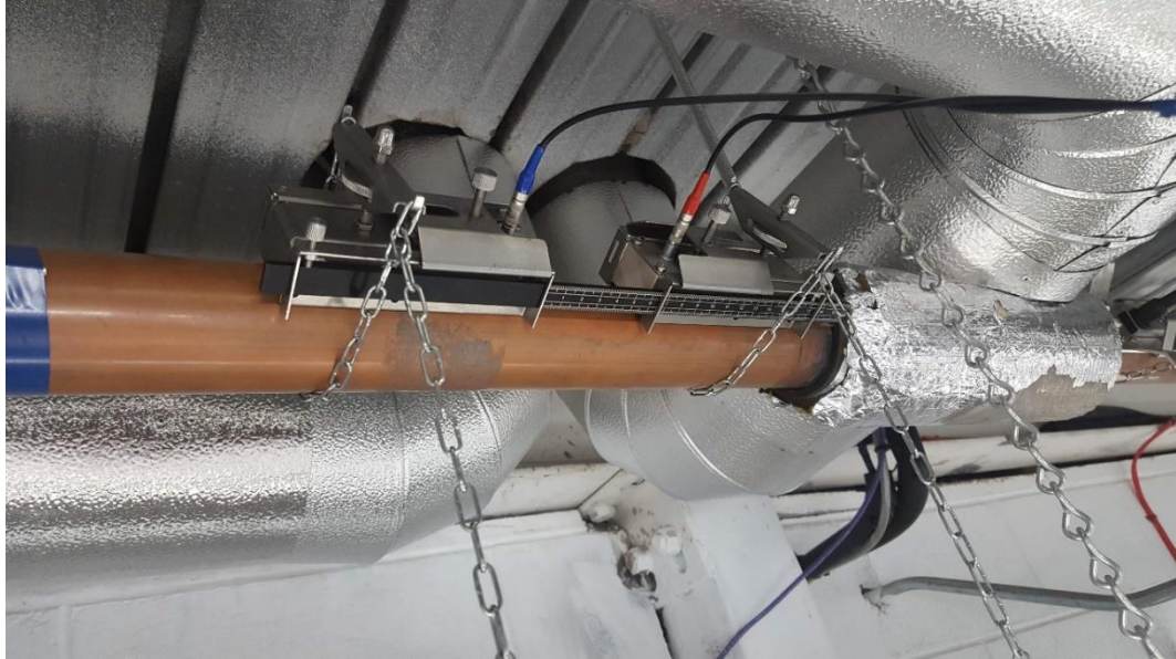
Figure 5-25 Installation of PF330 in the Postgraduate Centre
