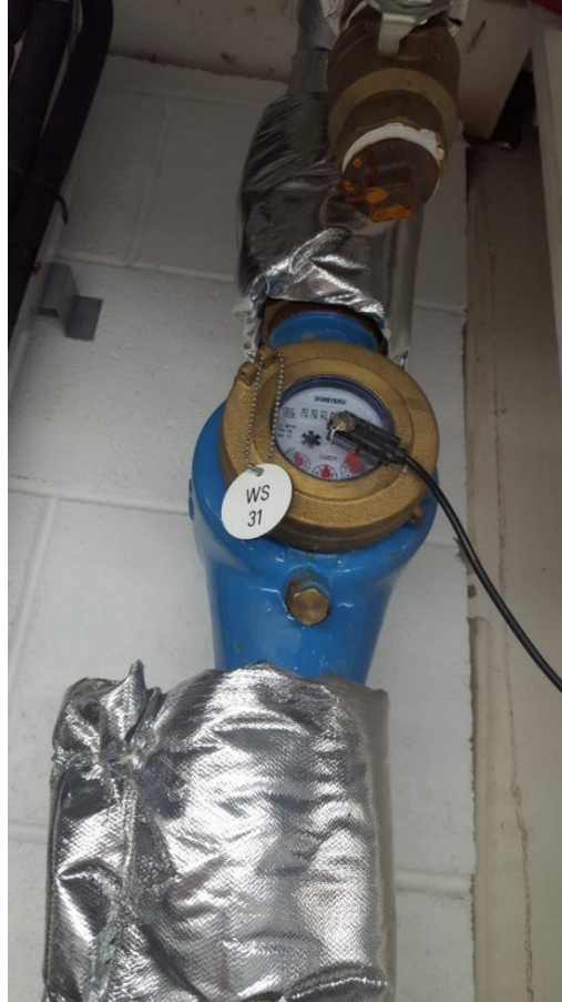
Figure 5-10 The fixed water meter in the Postgraduate Centre
