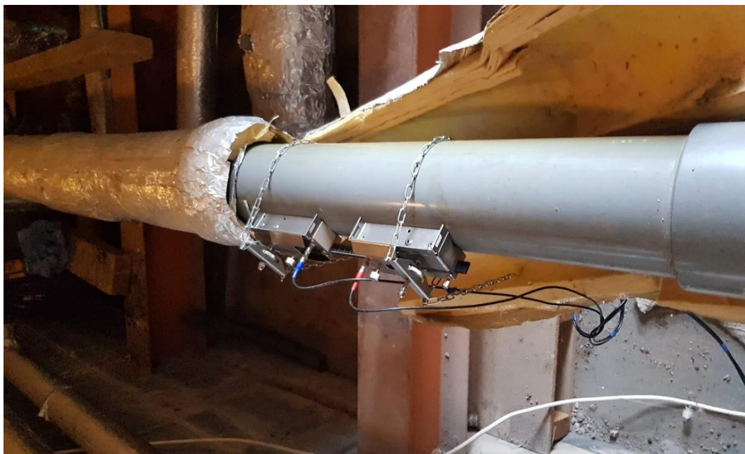
Figure 5-19 Installation of PF 330 in Estates building
