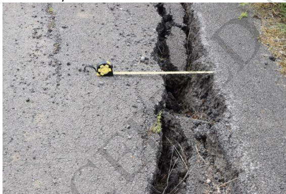
Figure 13 Longitudinal cracking at Witham Bank. Top: Superficial geology map. Bottom left: present day photograph (June, 2020). © Mark Heaton LCC. Bottom right: Road surface damage, looking south (May 2018) BGS © UKRI 2018
