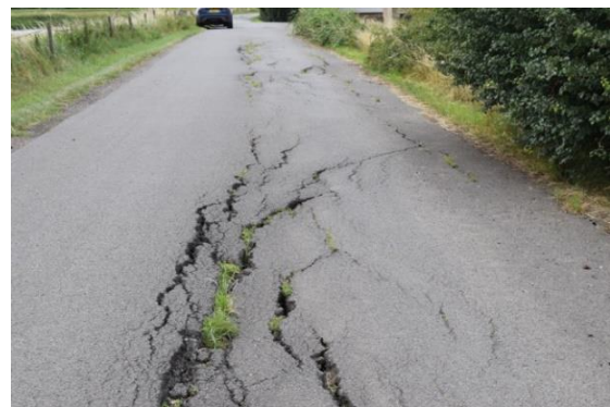
Figure 13 Longitudinal cracking at Witham Bank. Top: Superficial geology map. Bottom left: present day photograph (June, 2020). © Mark Heaton LCC. Bottom right: Road surface damage, looking south (May 2018) BGS © UKRI 2018
