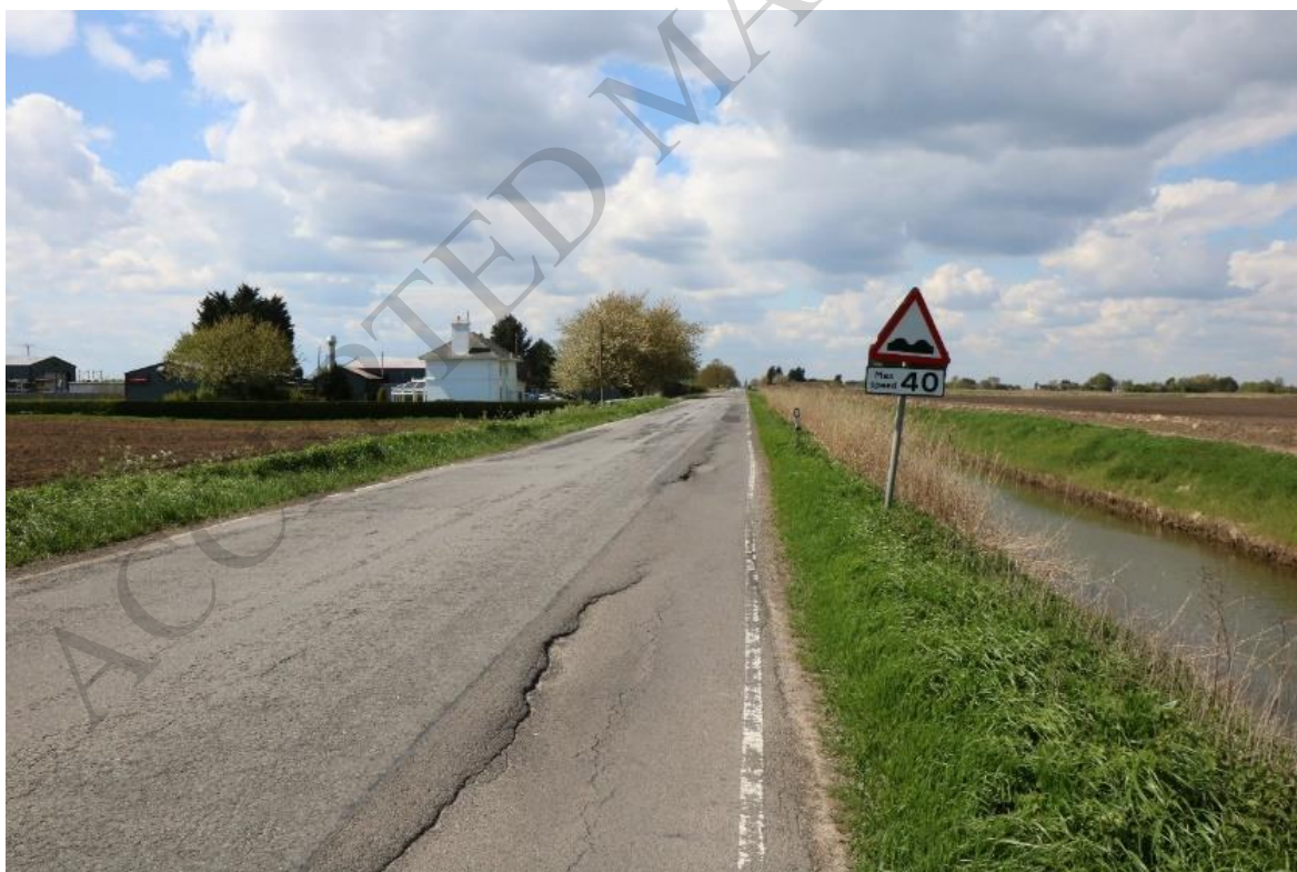
Figure 22 Station Road (Western end of Fodderdyke), Eastville, underlain by Tidal Flat deposits (May, 2018) BGS © UKRI 2018
