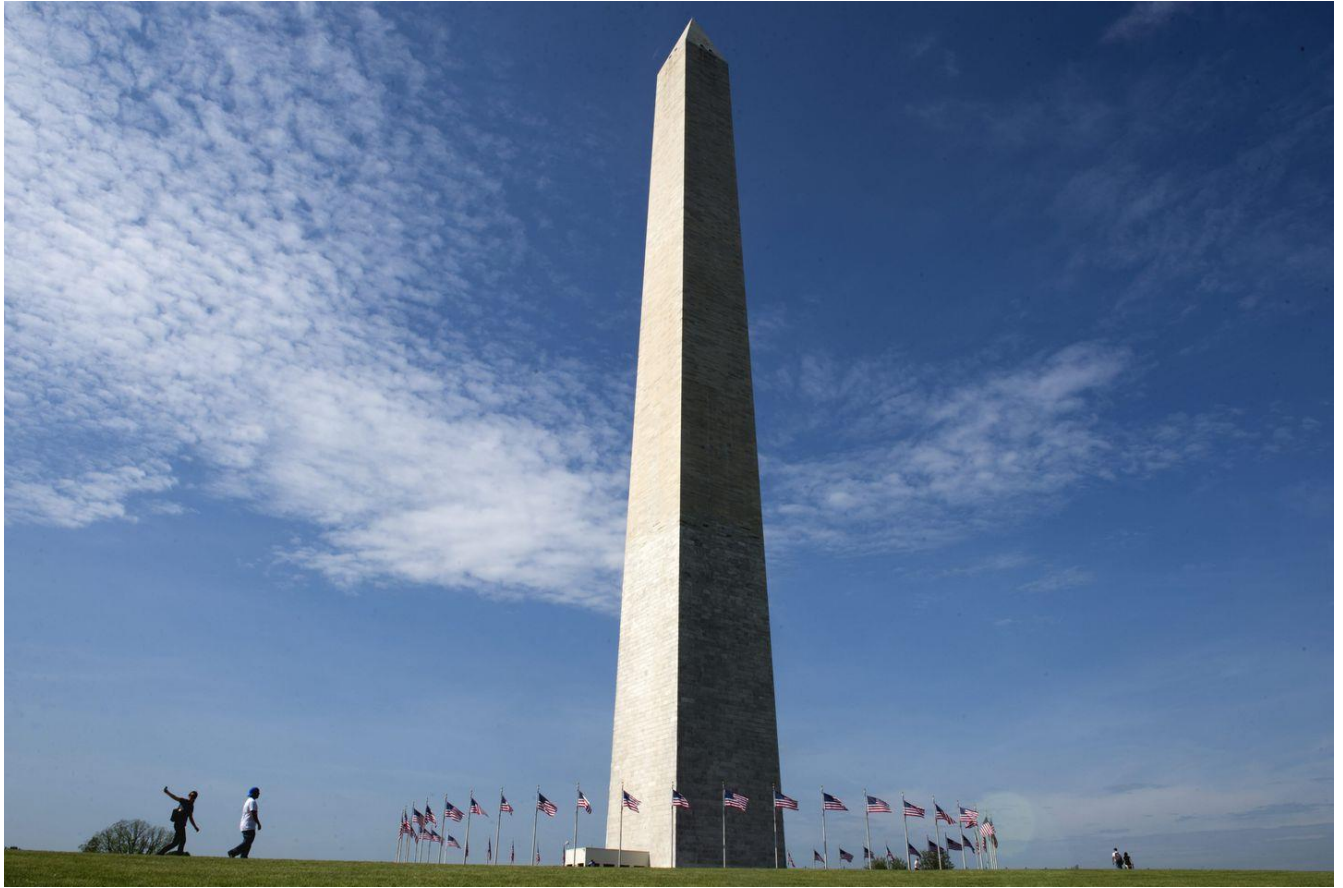
Figure 5.4 “Washington Monument Reopens After 2011 Earthquake.” BostonGlobe.com, 12 May 2014, www.bostonglobe.com/news/nation/2014/05/12/washington-monument-reopens-after-earthquake/7FWbZpx8fY8QVfYfmSFseO/story.html .
