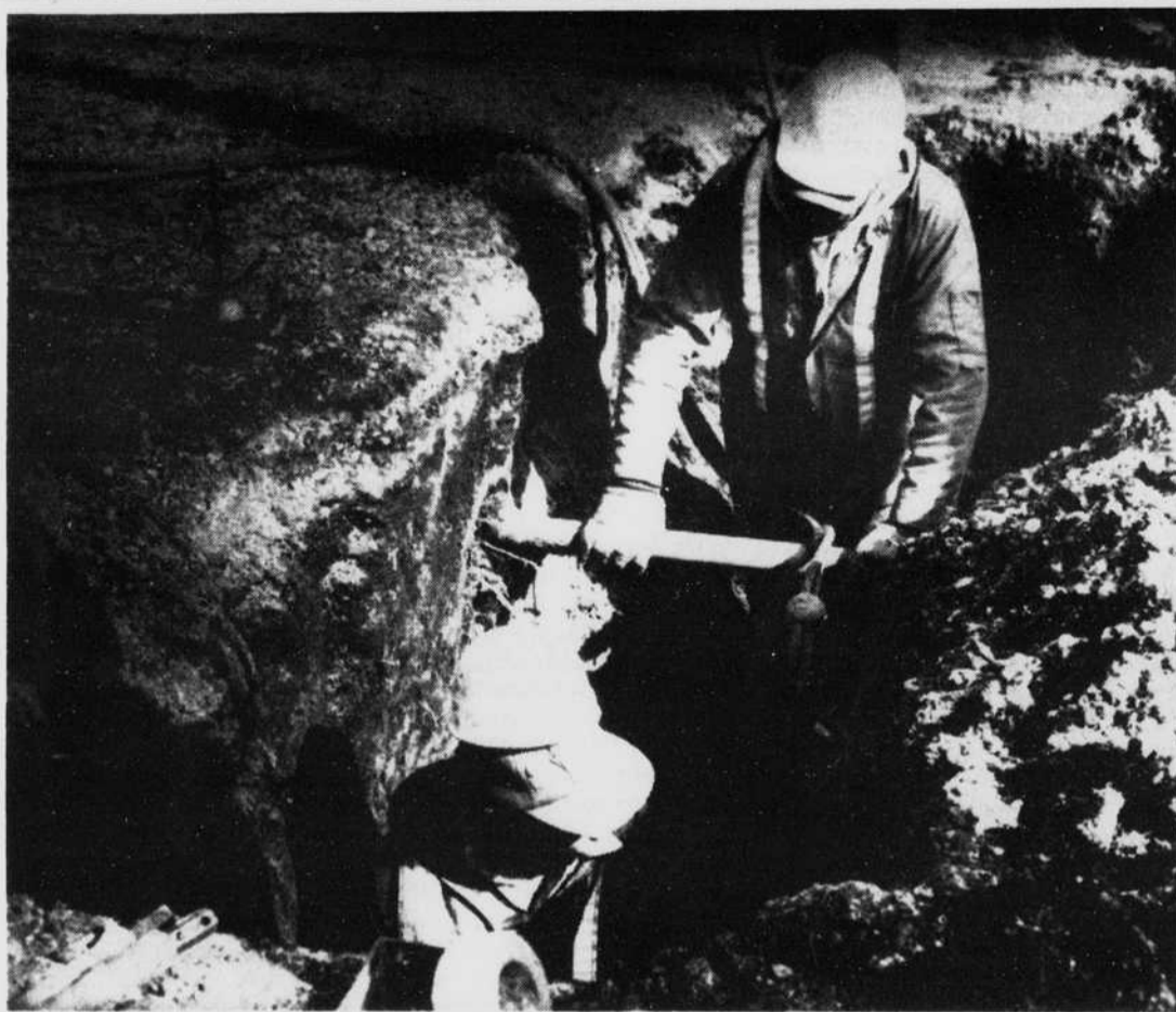
Larry Mennench (rear) and Terry Lawhead from Northern Illinois Water Corporation, install a two-inch main pipe near the Civil Engineering Building during Tuesday's unseasonably warm weather.
