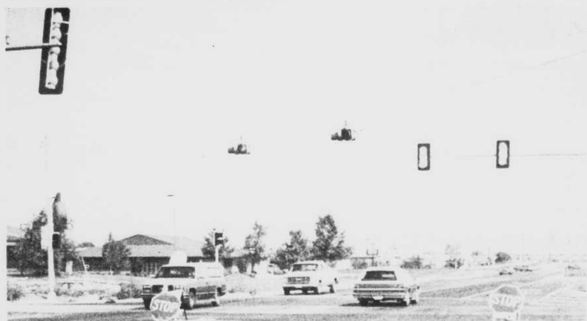
Work on the new traffic signal at the intersection of Country Fair Drive and University Avenue (I-72) in Champaign has been completed. Lights are tentatively scheduled to be turned on Sept. 11. Photo by Larry V. Gilbert
