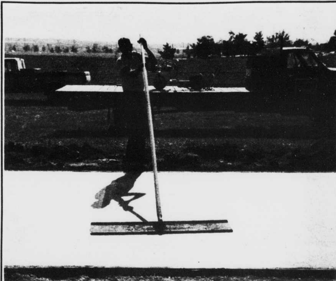
Smoothing the way -- Ray Luttrell, Pyramid Construction, Rantoul, is "bull floating" or mopping the concrete on Parkland Way Road.
