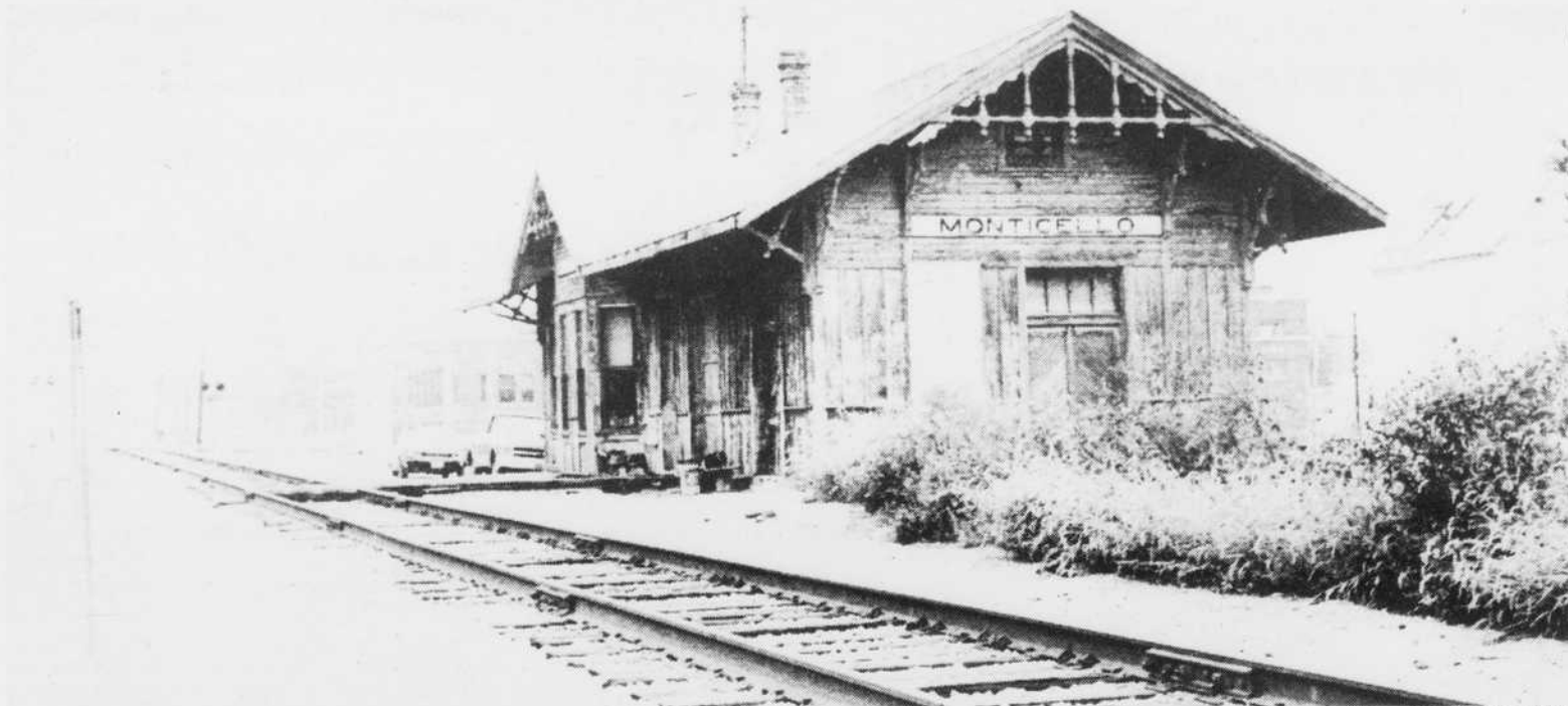
The old world charm of the now-abandoned railroad station is a reminder of the historic past to which Monticello can lay claim. Photo by Bridget Rund
