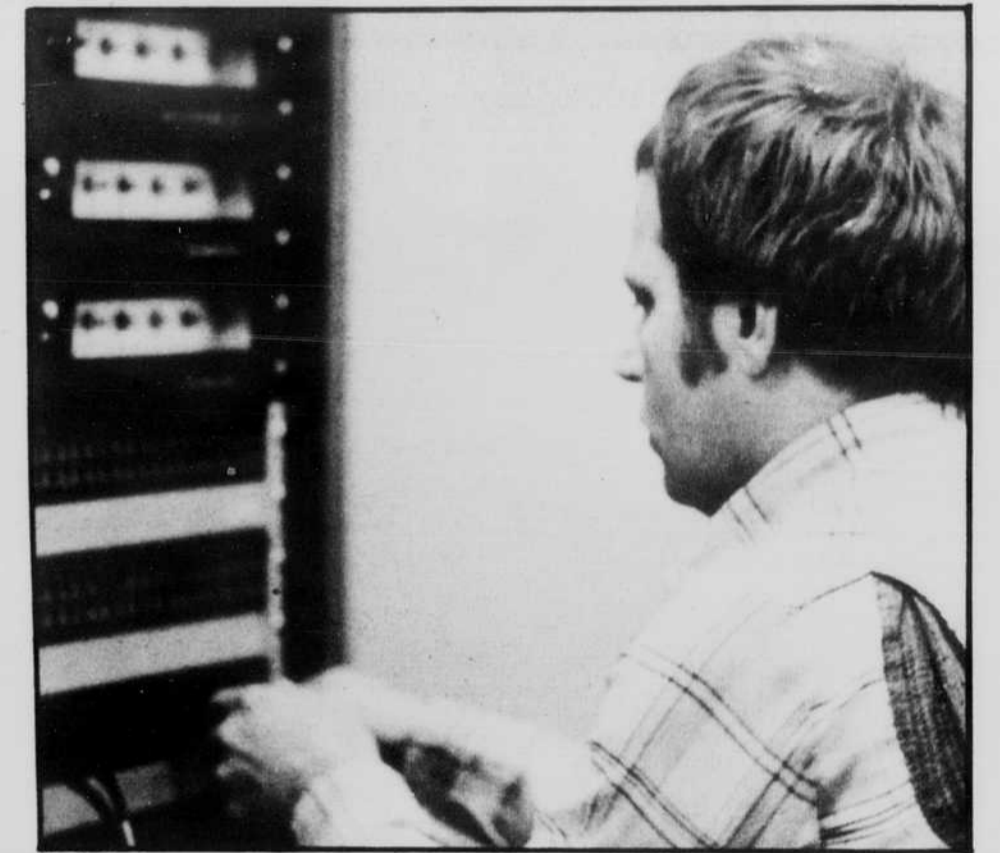
WPCD's Chief Engineer Ed Fiscus tests one of the patch bays as part final tests before going on the air.
