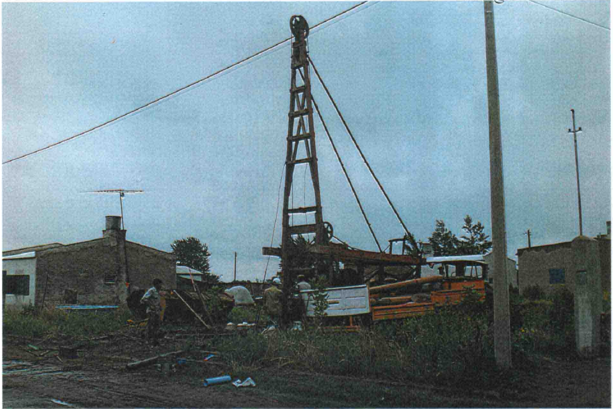
Plate 5.1 Talleres Norte drilling site, Eduardo Castex
