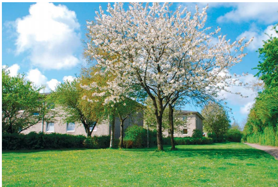
Figure 15. Photo of the apartment block. From http://www.kildeparken2020.dk (with permission).
