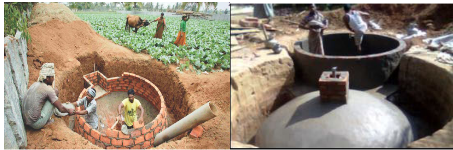
Figure 7. Sand Cement Brick—Fixed dome anaerobic digester Bangladesh.
