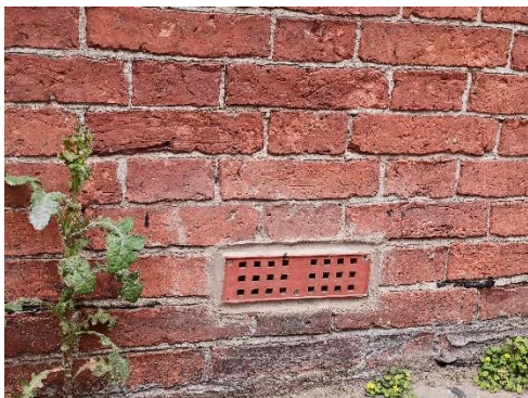
Photo 49 Air vent on the wall
