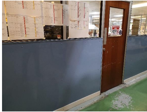
Photo 2 Plastic board on partition walls
