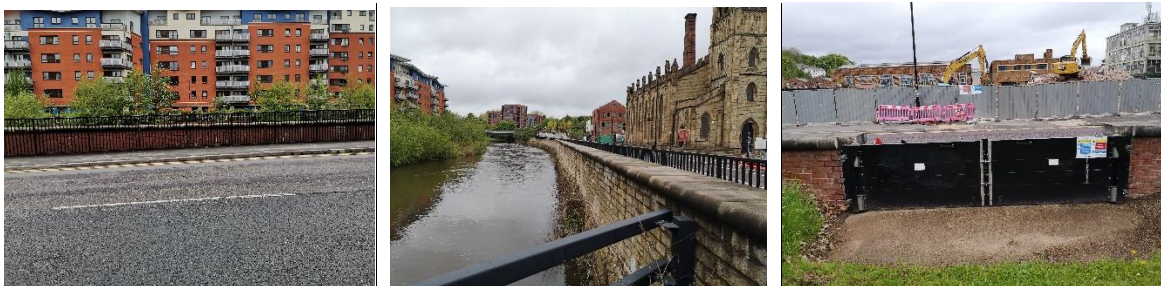
Photo 13/14/15 Flood defence wall along the river
