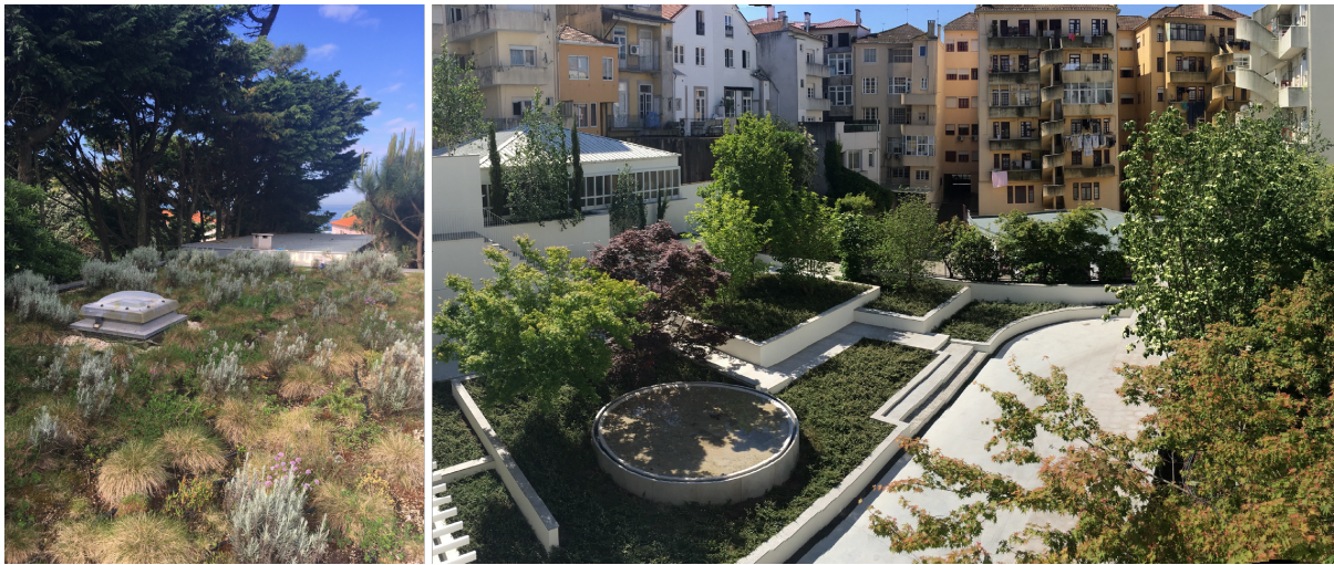
Figure 1. a) left side: extensive green roof and b) right side: intensive green roof (Porto, Portugal)
