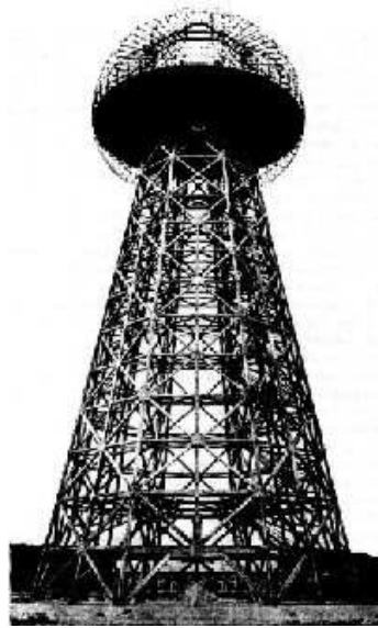
Figure 2.2: The 57 meters tall Wardencliff Tower (Mohammed et al., 2010).
