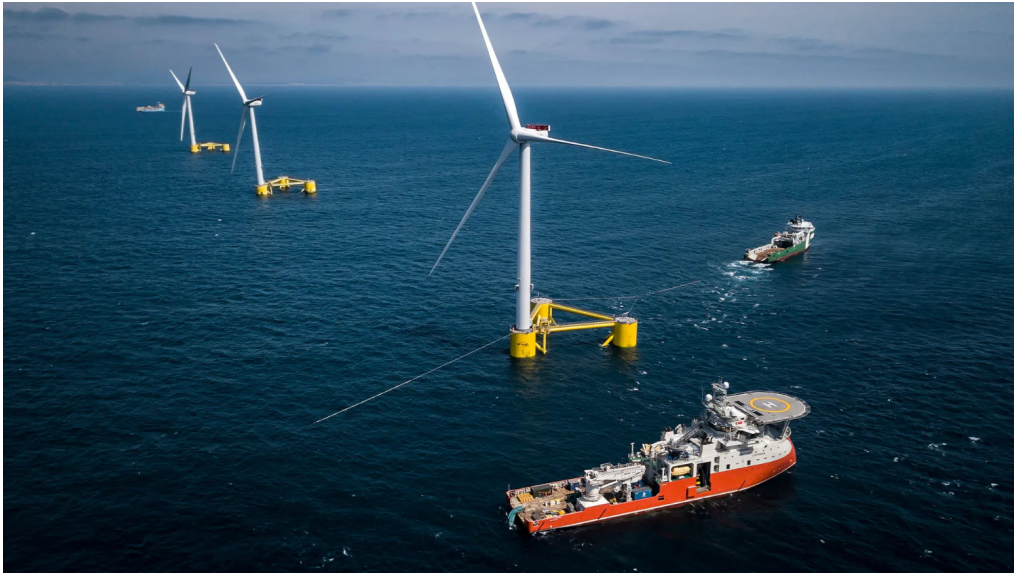
Figure 2.9: WindFloat Atlantic (Viana do Castelo, Portugal)
