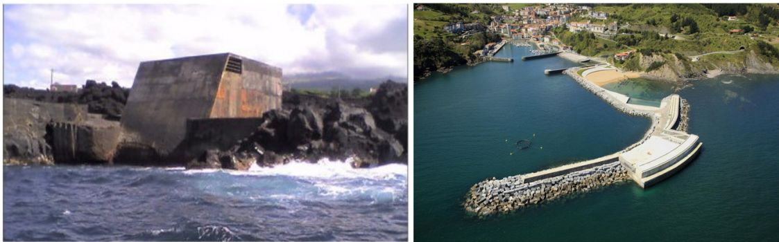
Figure 2.1: Pico plant, view from the sea (left); and Mutriku breakwater-mounted OWC (right).
