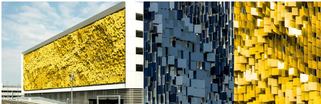
Figure 65. Urbana Architecture (2012). Dynamic facade system , Eskenazi Hospital Parking Garage, Indianapolis, USA
