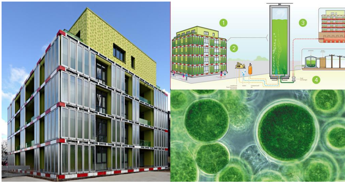
Figure 62. Splitterwerk, Arup GmbH, B+G Engineers, Immosolar (2013). The Bio Intelligent Quotient (B.I.Q.) Building, Hamburg, Germany
