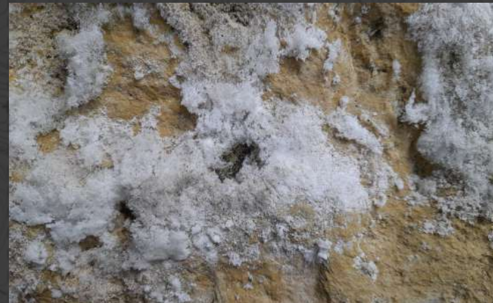
Efflorescences on the walls (elevation 13cm)
