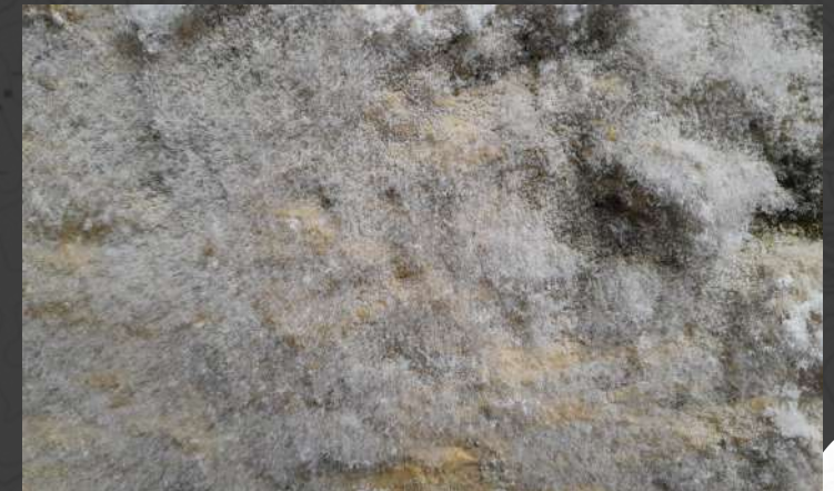
Efflorescences on the walls (elevation 13cm)
