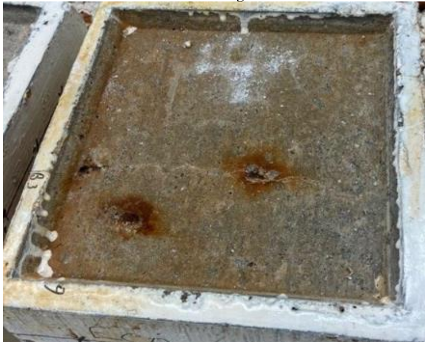
Figure 3.56: Surface staining on Southern Exposure specimen with conventional reinforcement
